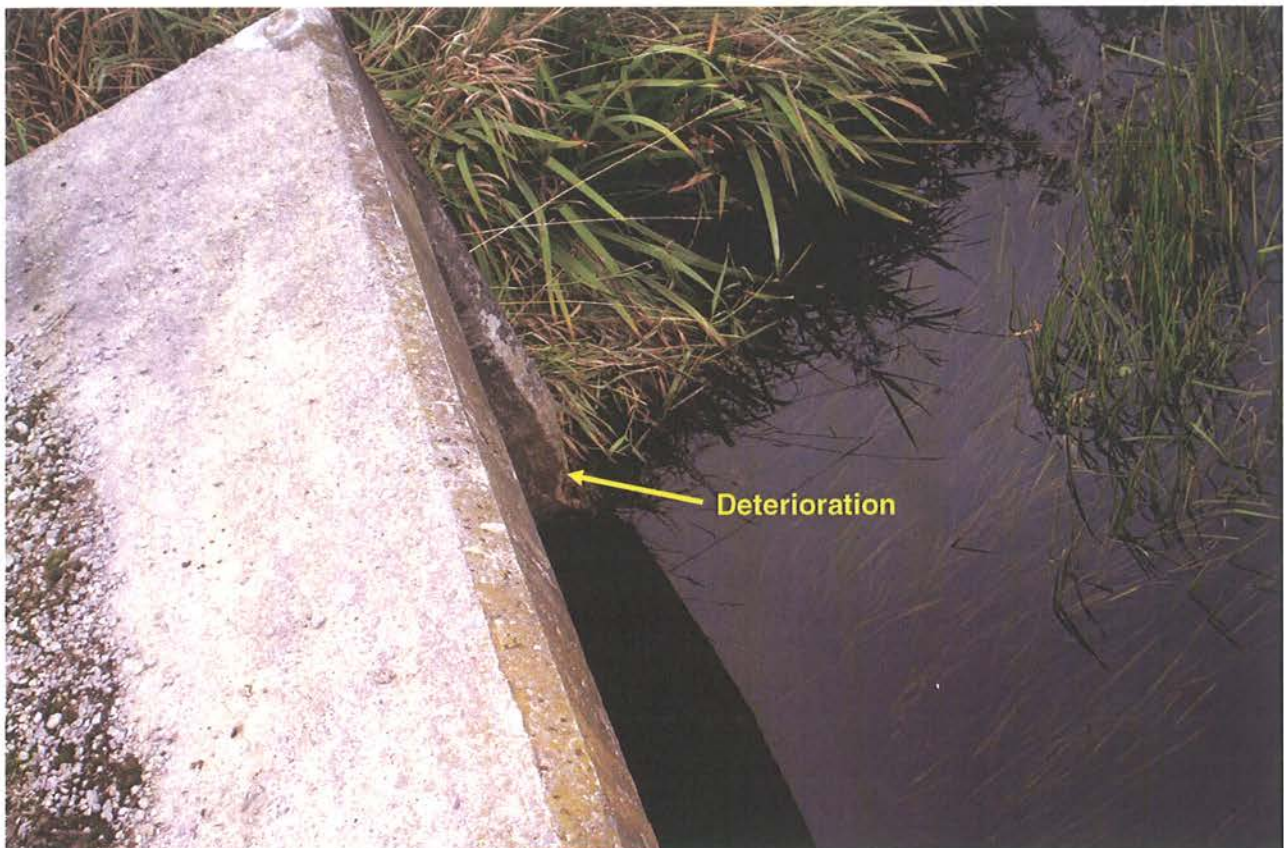
Photo No. 4: Culvert at outlet showing signs of deterioration
