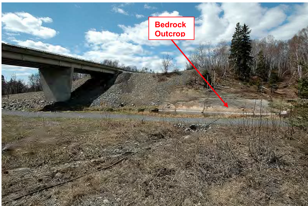
Photograph 2: Looking west from proposed east abutment location. Note bedrock outcrop at west pier location. (May 2, 2007)
