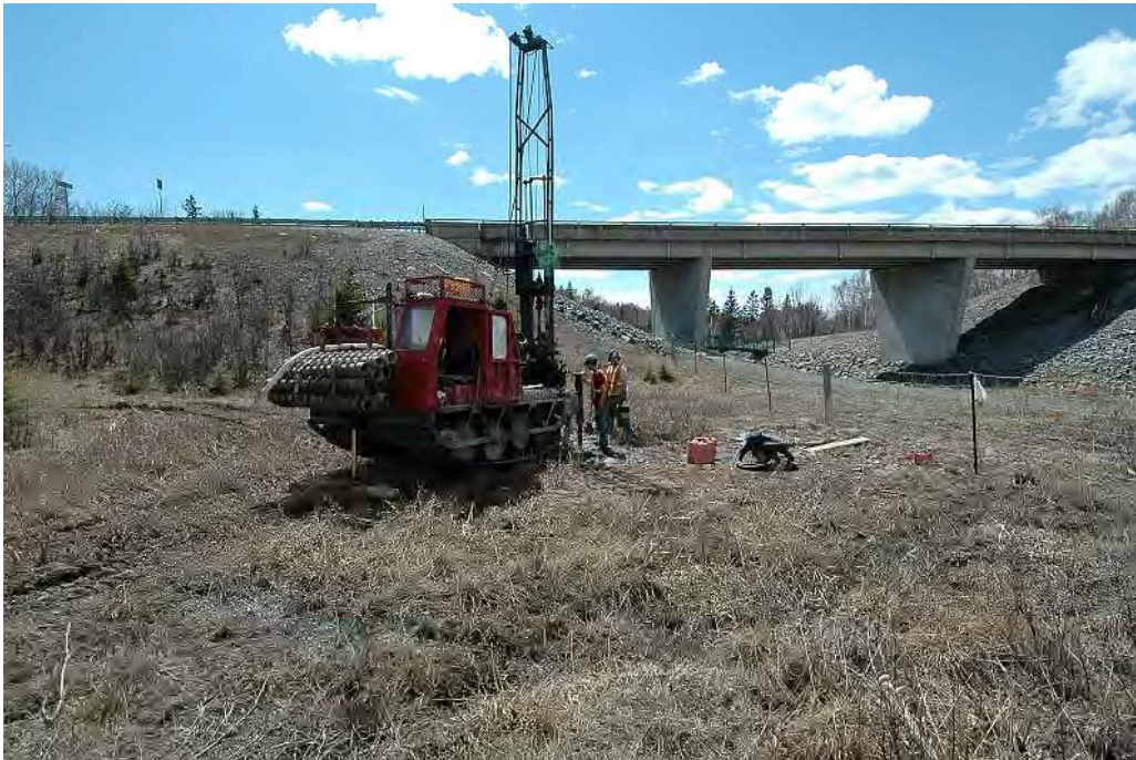
Photograph 1: Looking southwest from east of the structure site. Drill rig at borehole L1-2 (proposed east abutment location). (May 2, 2007)
