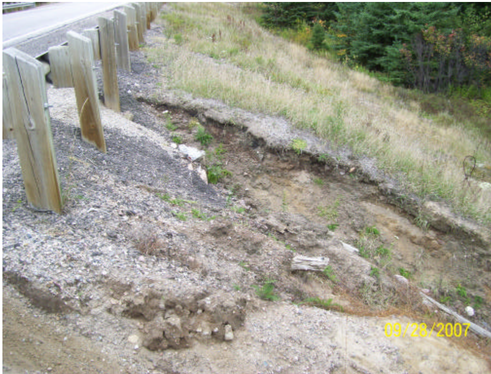
Photograph 5. Surficial erosion at Resmer Creek Culvert location
