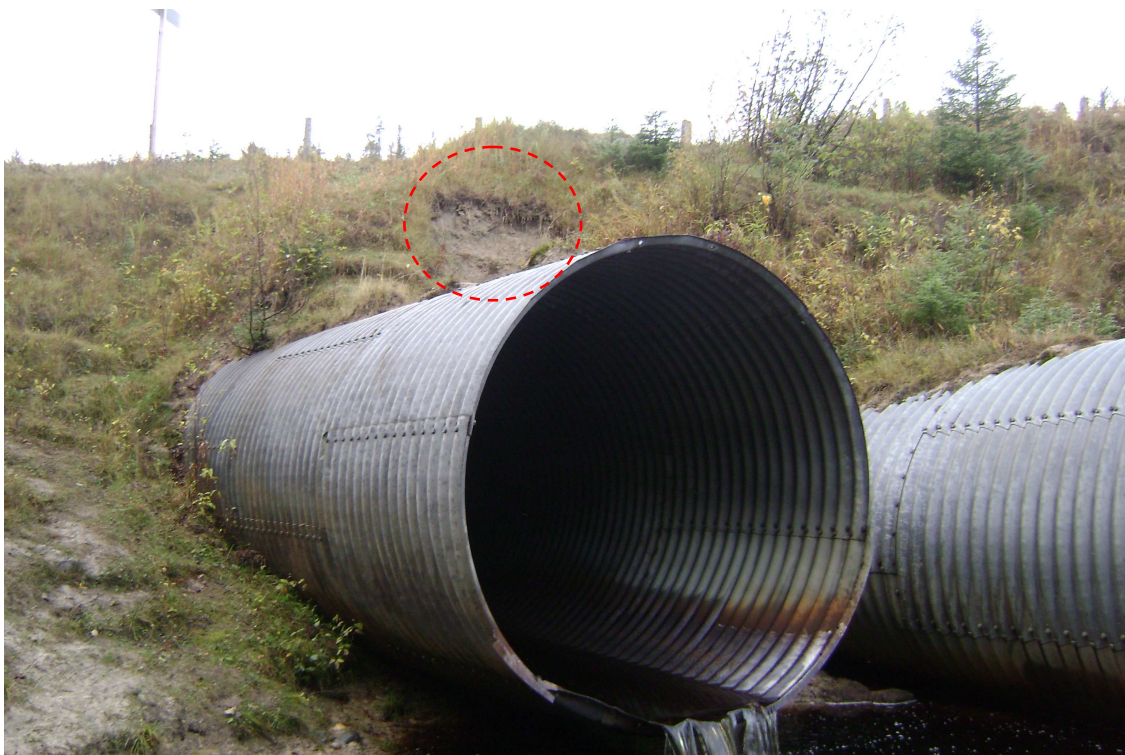
Photograph 3 East side of Embankment showing erosion of slope
