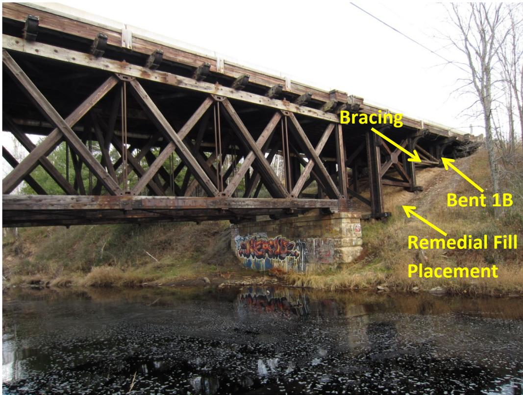
Photo No. 3: East bridge pier, looking northeast
