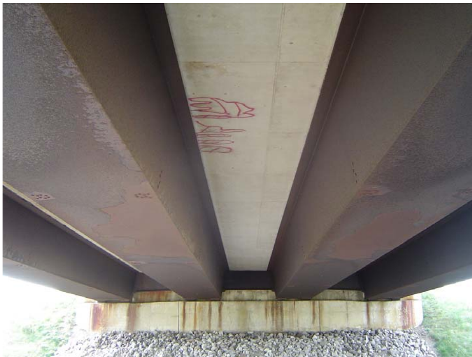
Photo 8: General view of soffit over eastbound lanes, looking towards the south abutment. Rip-rap slope protection is visible at bottom of photograph.
