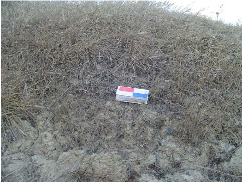
Photo 7: Tension cracks near top of south face of northwest approach fill.
