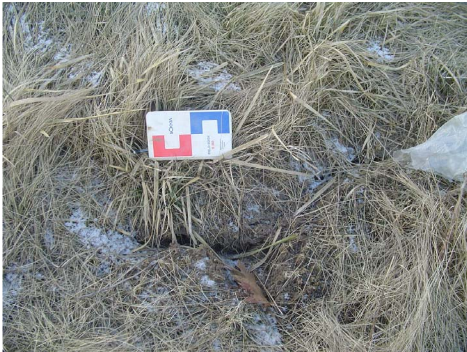
Photo 3: Tension crack along southwest approach fill.
