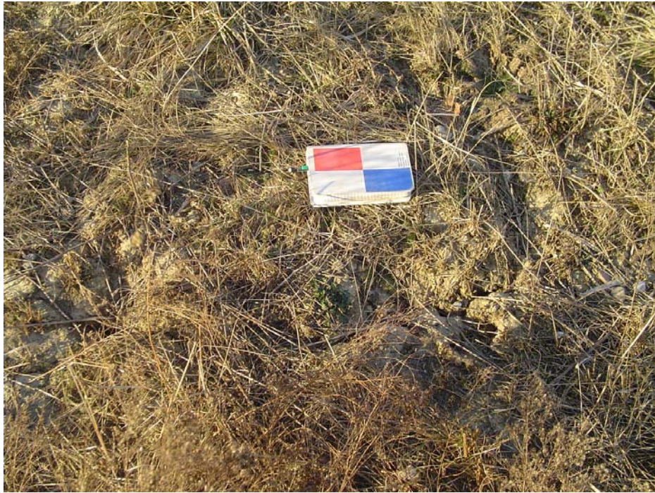
Photo 5: Tension cracks near toe of south face of northwest approach fill.
