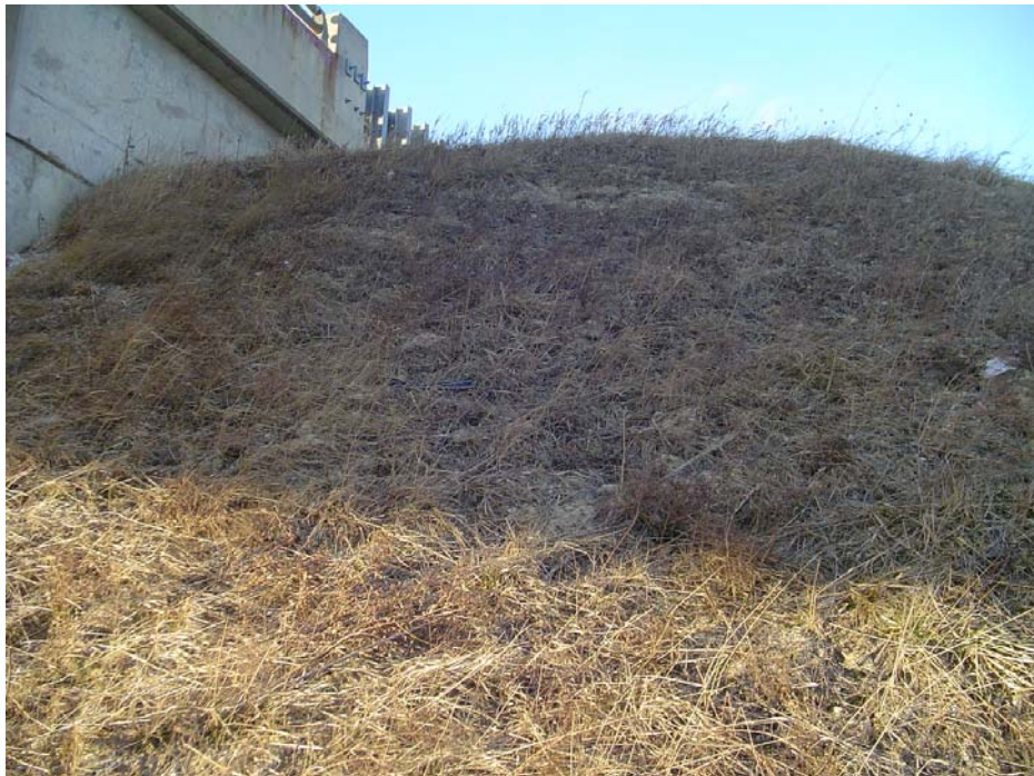
Photo 6: Loss of vegetation on south face of northwest approach fill.
