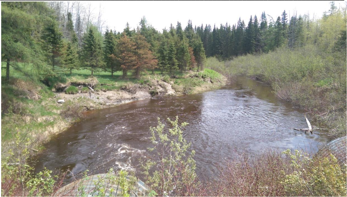
Photo 3: Looking east from Culvert North Barrel Outlet. Slope erosion visible on north bank of creek
