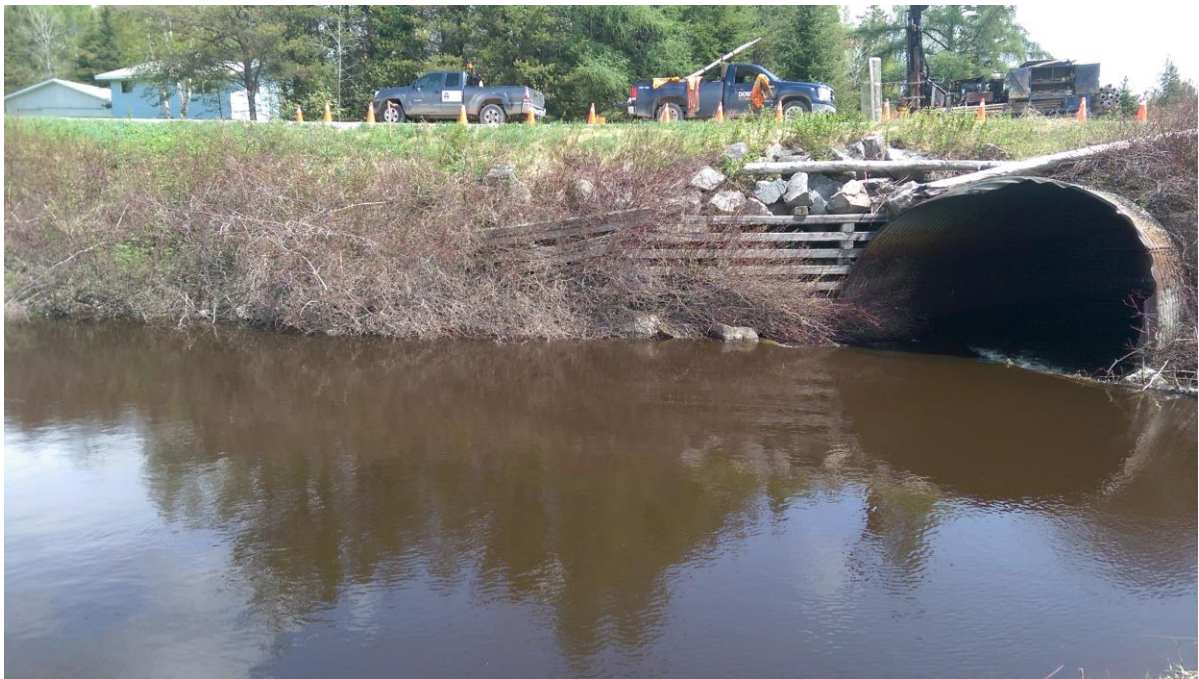
Photo 4: Looking East towards Culvert North Barrel Inlet. Retaining Structure with Rock Fill noted along road embankment.
