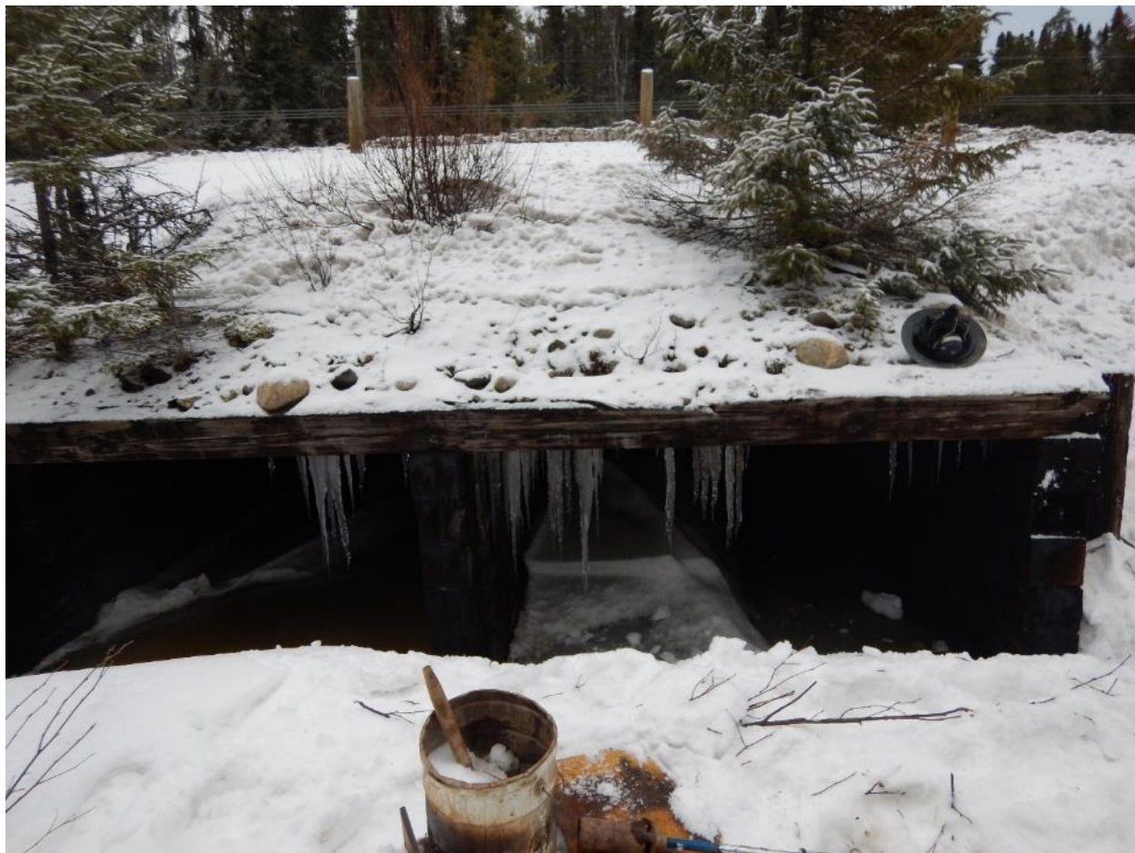
Photo 4: Wawiag Creek Culvert, south side – timber cells
