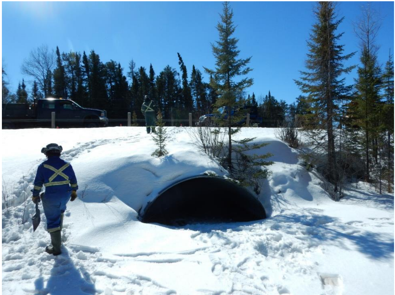
Photo 3: Wawiag Creek Culvert, north side – CSP extension
