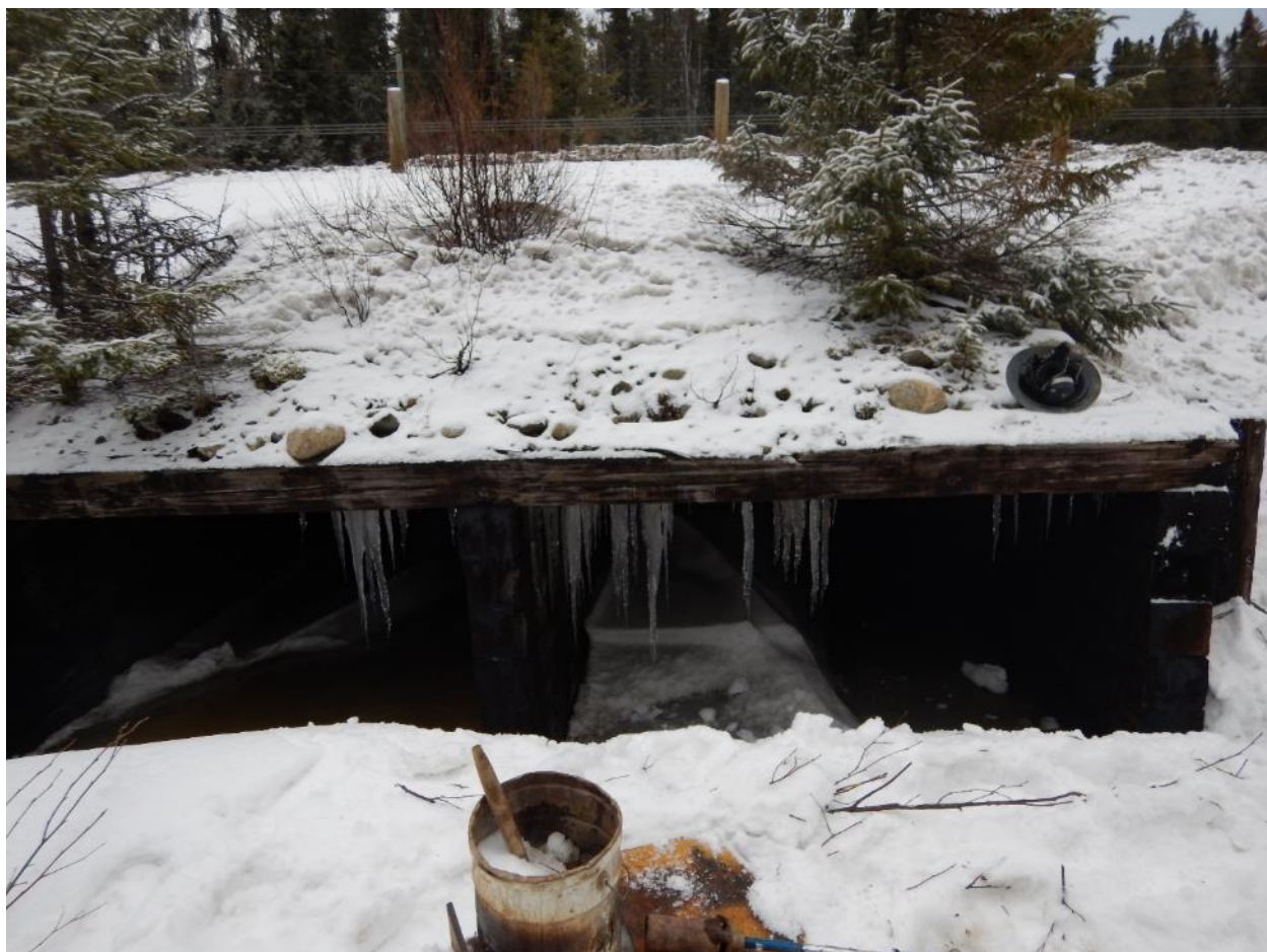
Photo 4: Wawiag Creek Culvert, south side – timber cells
