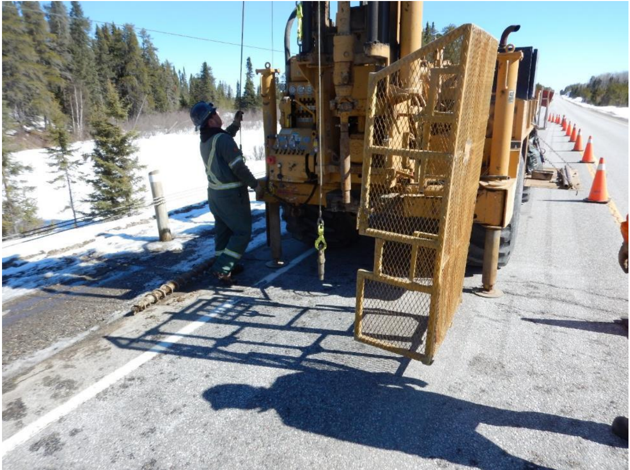
Photo 2: Highway 11 embankment over Wawiag Creek Culvert, facing east – drill rig setting up
