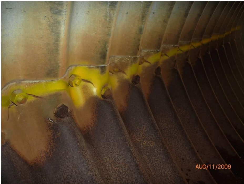
Figure 2.4 Failure at culvert connections
