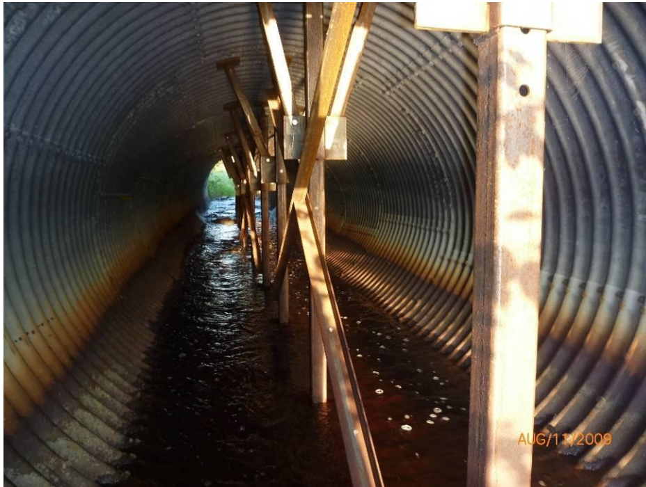
Figure 2.3 Culvert supports
