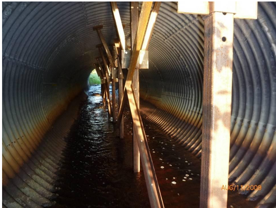
Figure 2.3 Culvert supports
