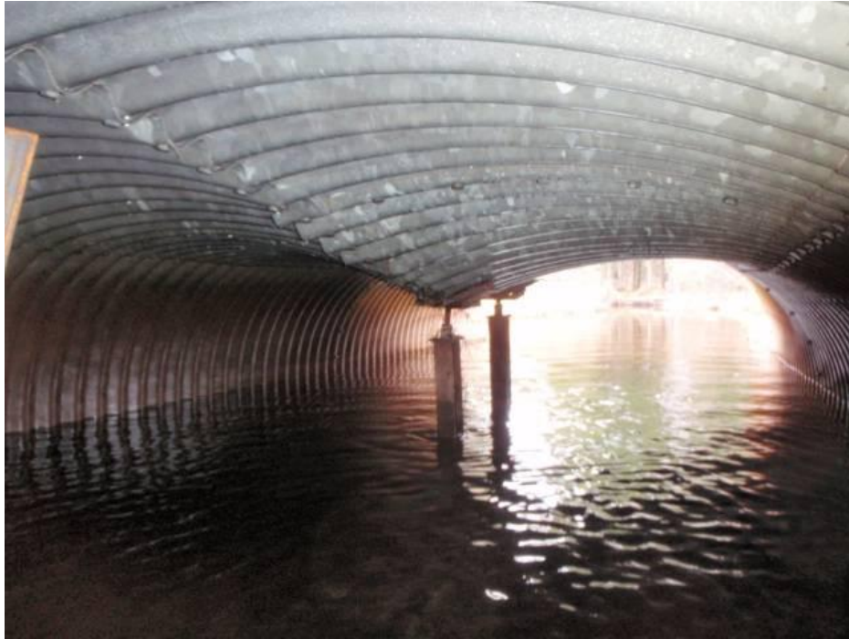
Figure 2.3 Culvert supports
