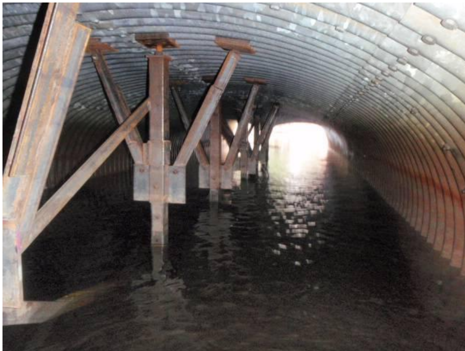
Figure 2.4 Additional culvert supports
