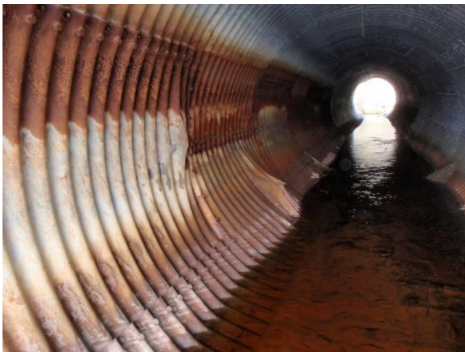
Figure 2.4 Culvert buckling
