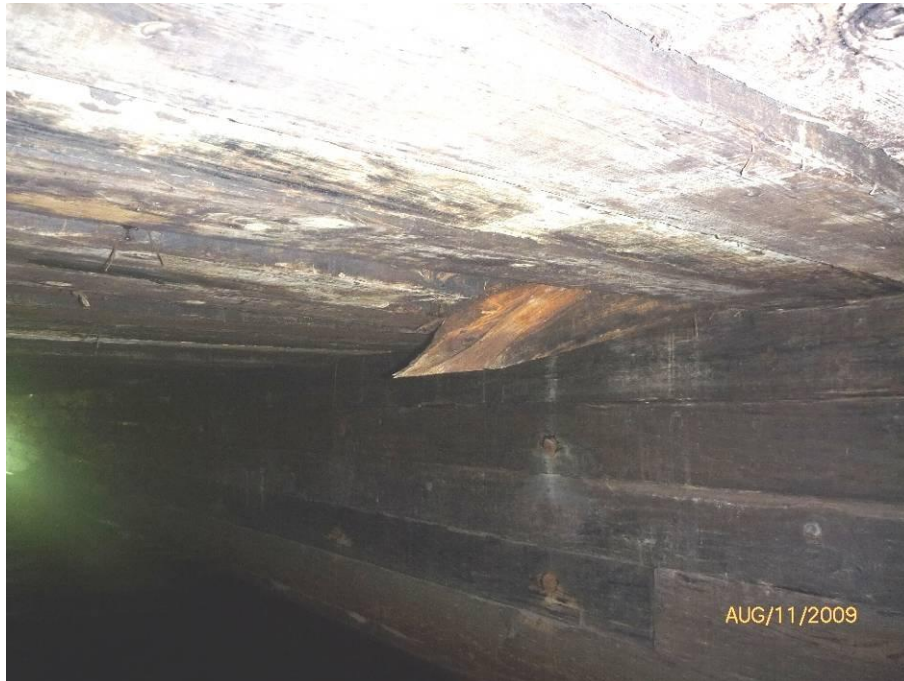
Figure 2.3 Culvert deterioration
