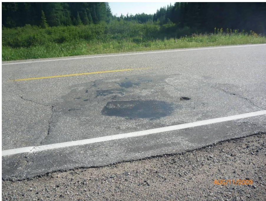
Figure 2.8 Asphalt deterioration facing northeast
