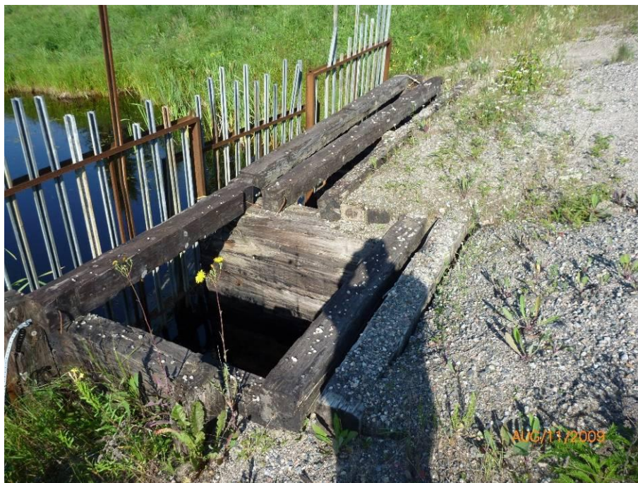
Figure 2.4 Missing culvert sections
