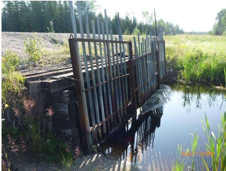
Figure 2.1 Culvert inlet (facing northeast)
