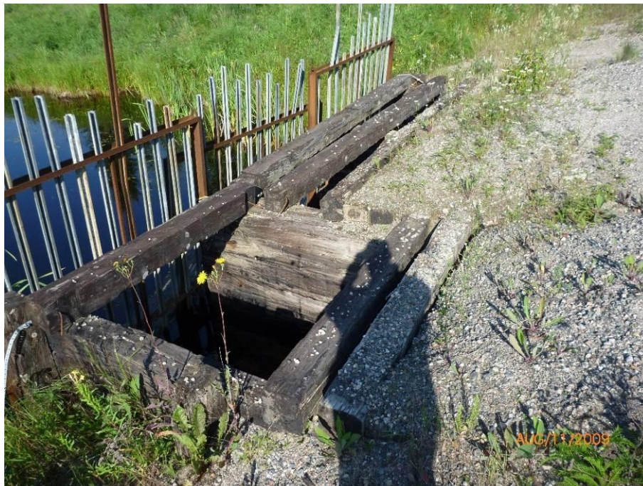
Figure 2.4 Missing culvert sections
