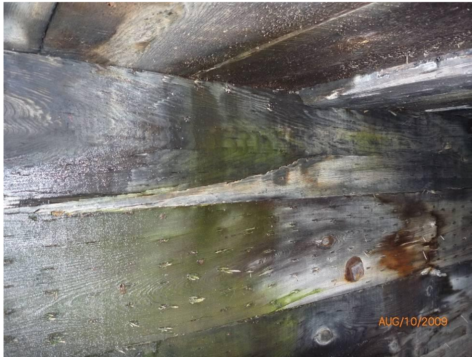
Figure 2.4 Culvert Deteriorating
