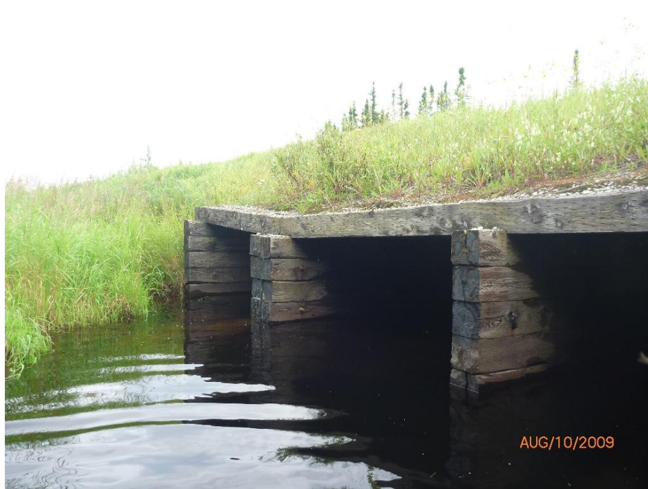
Figure 2.3 Culvert Buckling
