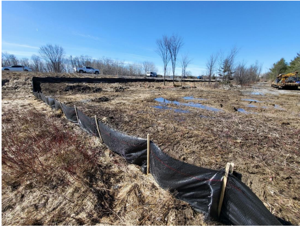
Photo 5. Looking southwest along silt fence near to the culvert site (March 12, 2024)
