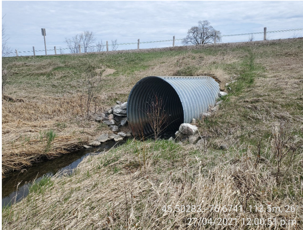
Photo 3. Culvert inlet (2021/04/27)
