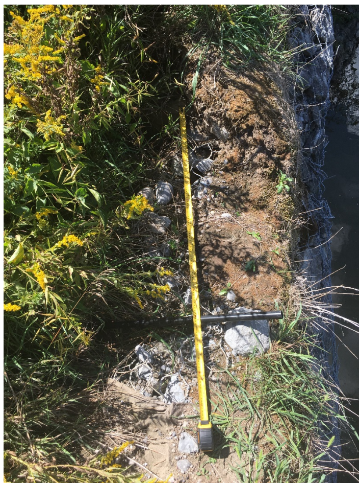
Photograph B3: No Geotextile Fabric Visible Behind Wall – Looking West Along Top of Wall
