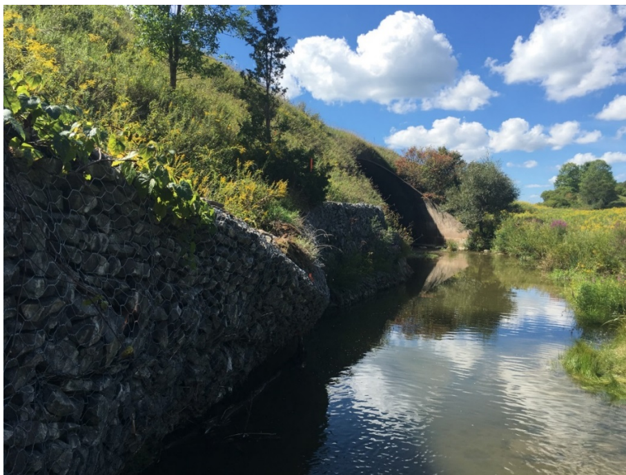
Photograph B2: Translation/Toppling of Gabion Basket Retaining Wall – Looking West
