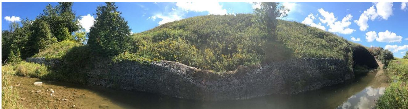
Photograph B1: Deformed Area of Gabion Basket Retaining Wall – Looking South (Note image distortion due to panoramic view)
