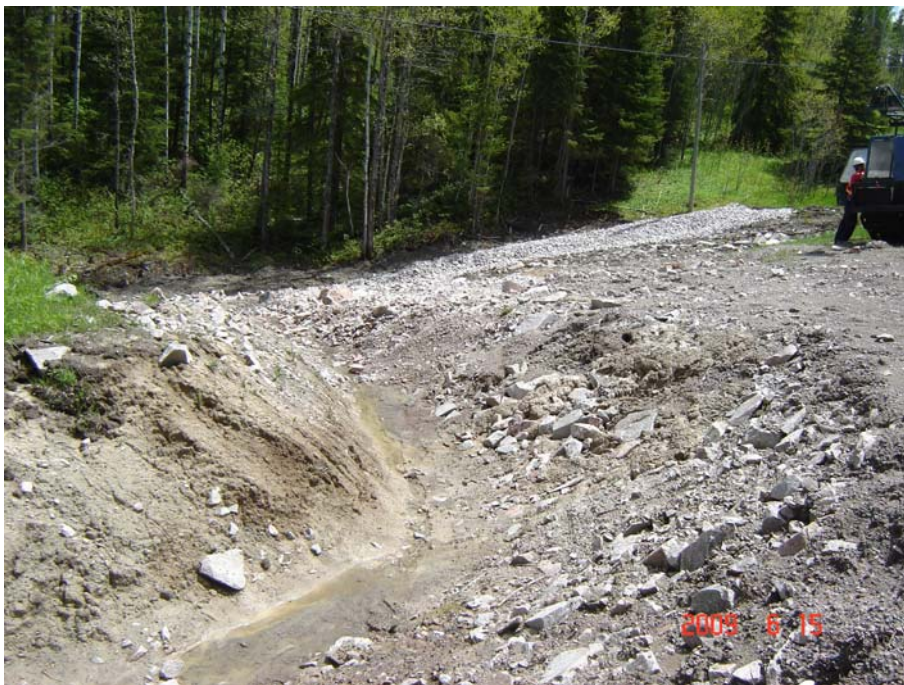
Photograph 4: Culvert # 60 at Station 11+684 (Pacaud Township). On east side of Highway 11, looking south-east. Failed slope and north roadside ditch.
