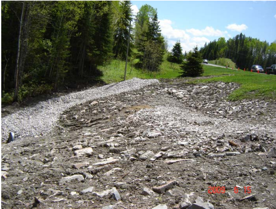
Photograph 3: Culvert # 60 at Station 11+684 (Pacaud Township). On east side of Highway 11, looking south. Culvert outlet and gravel lined ditch.
