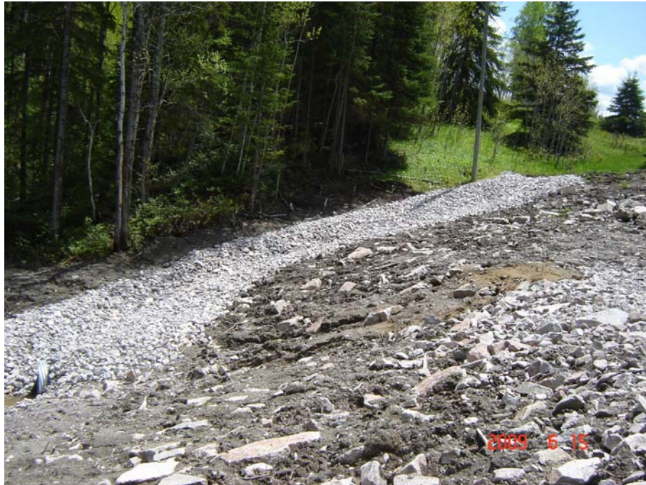
Photograph 5: Culvert # 60 at Station 11+684 (Pacaud Township). On east side of Highway 11, looking south. Culvert outlet and gravel lined ditch.
