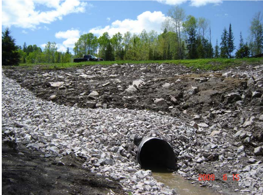
Photograph 1: Culvert # 60 at Station 11+684 (Pacaud Township). On east side of Highway 11, looking west. Culvert outlet and failed CSP pipe.
