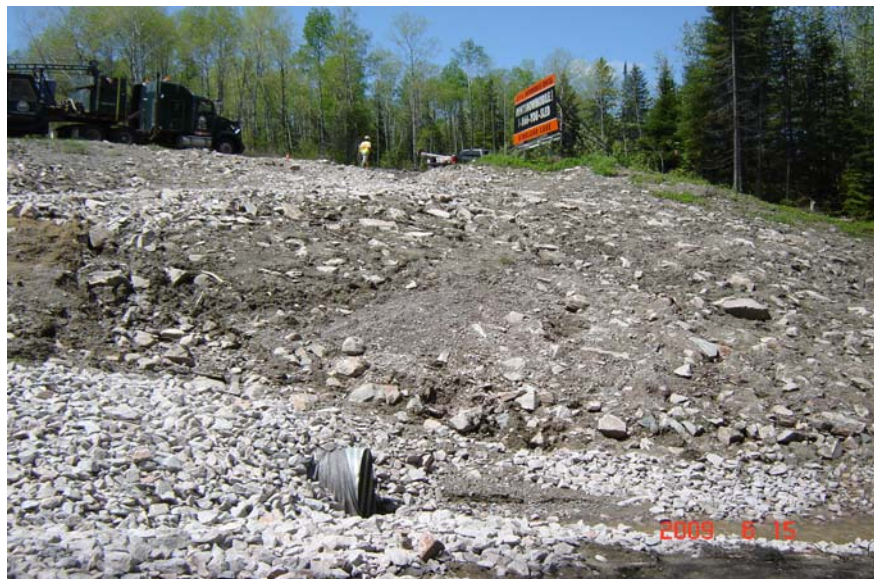
Photograph 2: Culvert # 60 at Station 11+684 (Pacaud Township). On east side of Highway 11, looking north-west. Failed slope.
