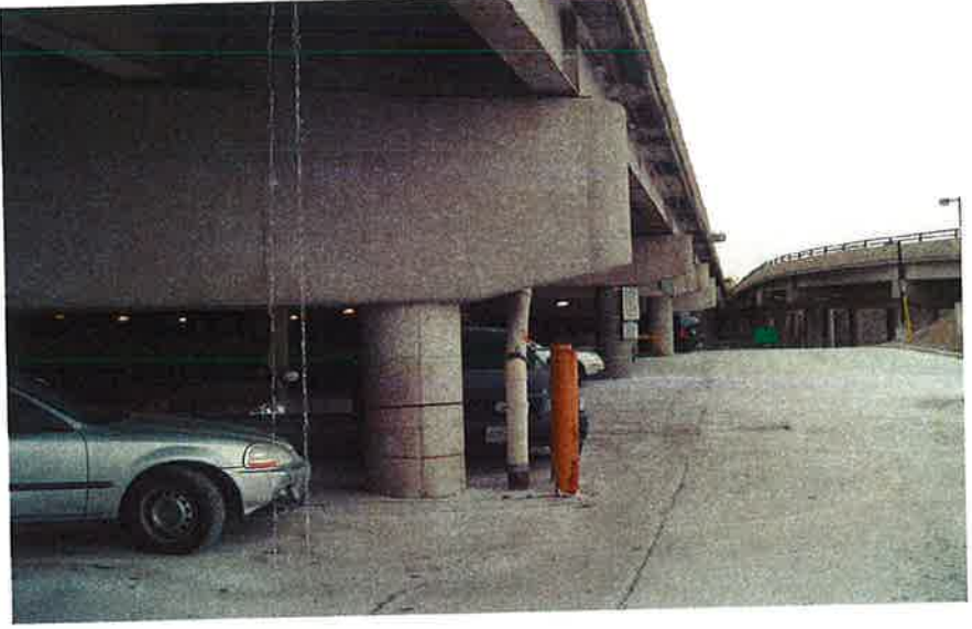
Photograph 6 View looking west, north end of Bent 126 through 123. Note difference in beam depths where repairs have been made.
