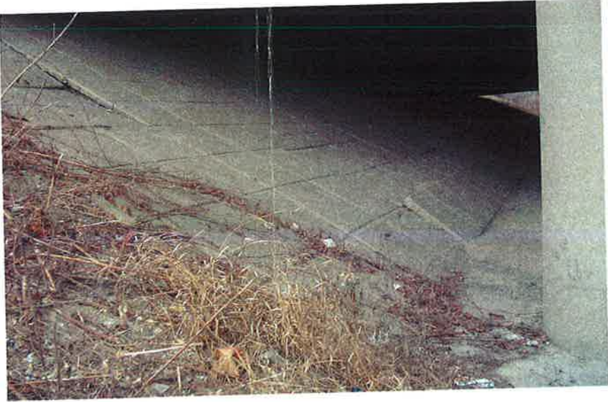
Photograph 5 North end of concrete paved slope, east of Leslie Street. Note displacement of concrete and evidence of migration of fines at toe.
