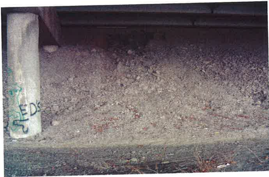
Photograph 1 Typical erosion noted below West Collector Lanes.
