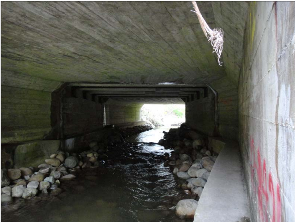
Photograph No. 2: View inside the culvert.
