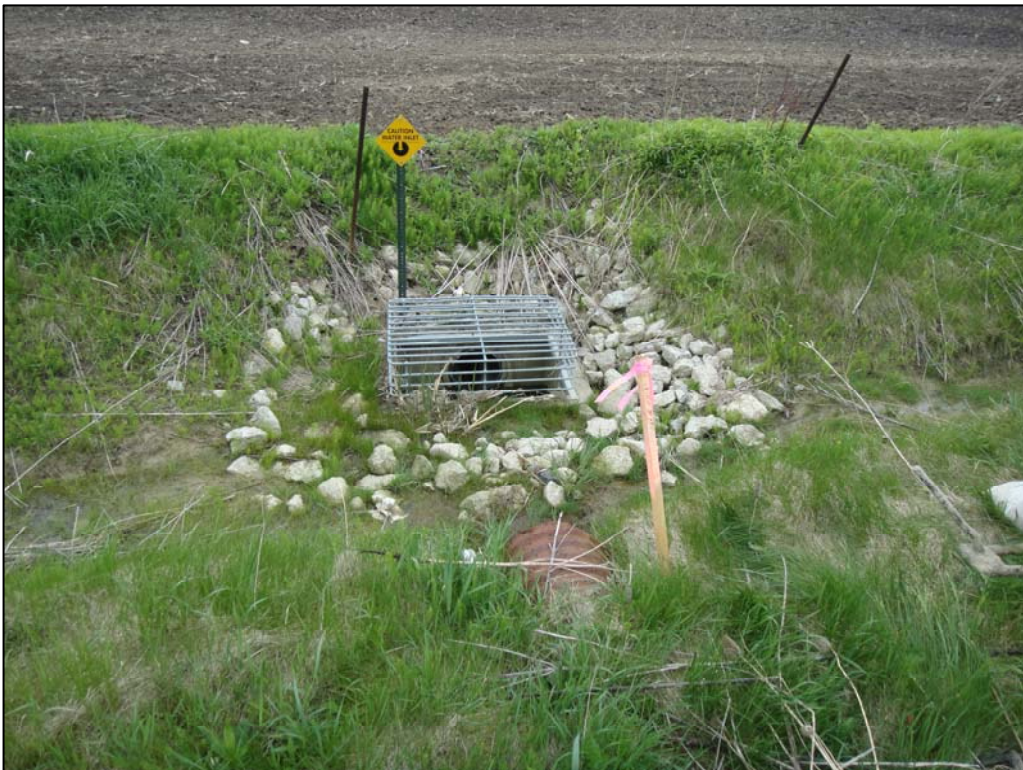
Photograph No. 2: View of culvert outlet.
