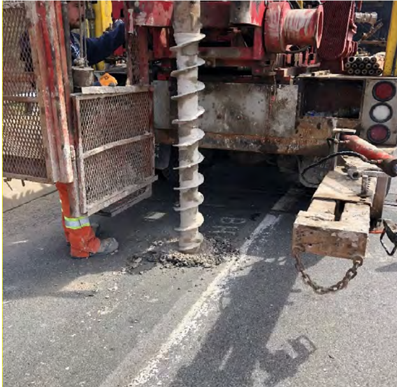
Photo 3: Looking west – Borehole drilling at 22-06 with truck-mount drill rig
