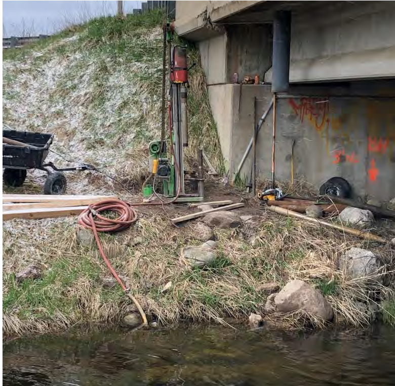
Photo 4: Looking west – Borehole drilling at 22-03 with portable Hilti drilling machine
