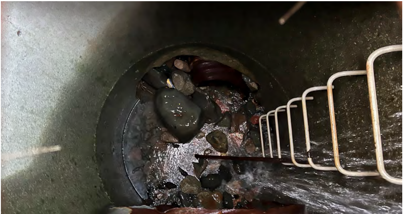
Photograph #4 – Cobbles and boulders inside drop inlet located along ditch line. (November 2022)
