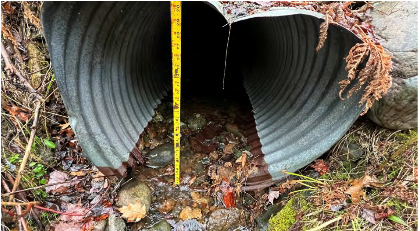
Photograph #5 – Partially crushed culvert outlet, facing south. (November 2022)
