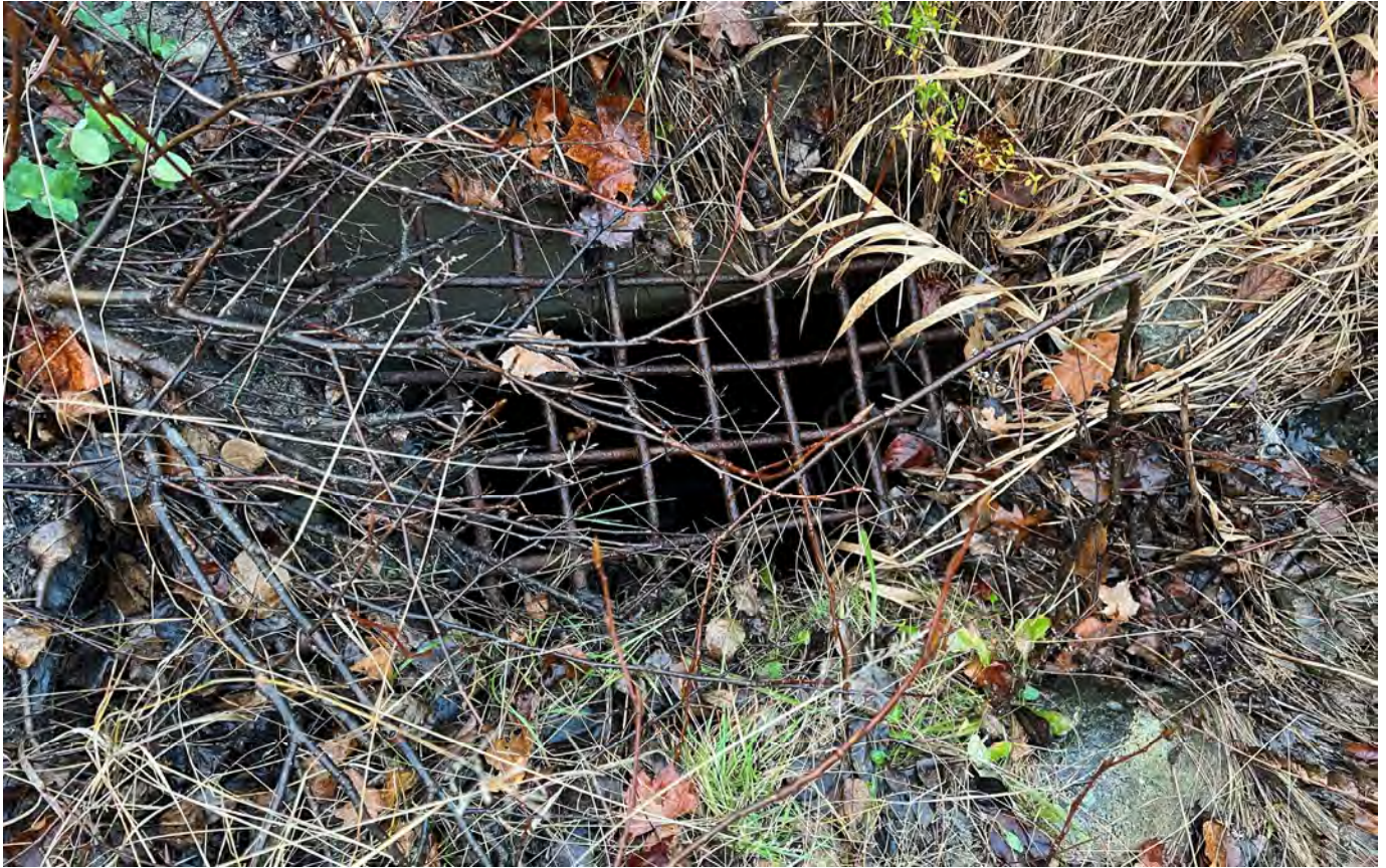
Photograph #3 – Safety grate over drop inlet at the culvert inlet located along ditch line. (November 2022)
