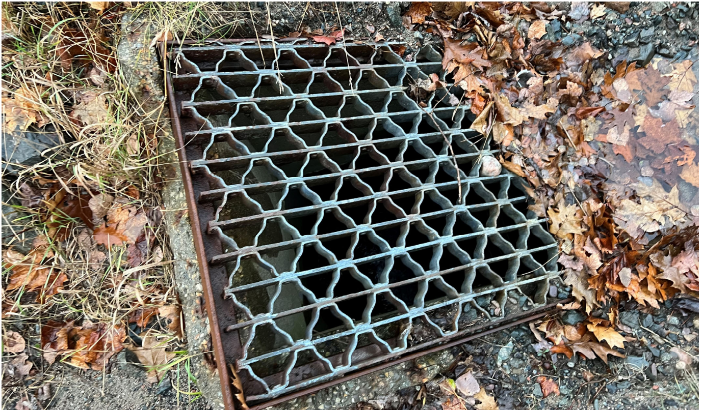
Photograph #3 – Safety grate over drop inlet at the culvert inlet (November 2022)
