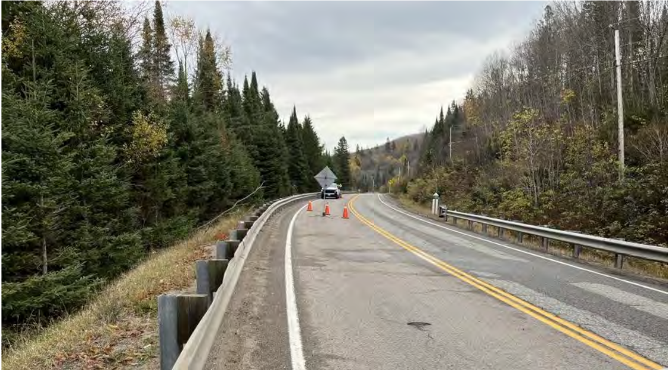
Photograph #1 – Highway 556 at STA 19+596, looking East. Embankment slope facing north is sparsely vegetated (October 2022)
