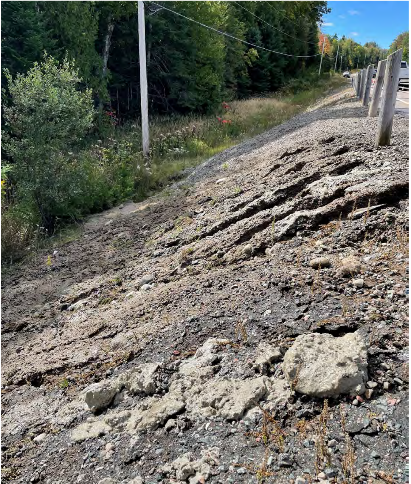
Photograph #5 – Surficial erosion of the unvegetated portion of the south-facing embankment slope, facing west.
