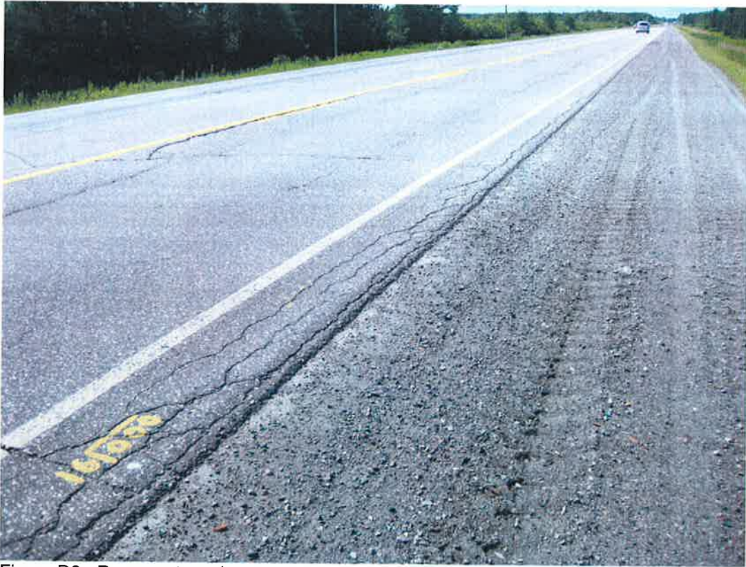
Figure D3 - Pavement cracks at Passing Lane 4, about Station 16+000
