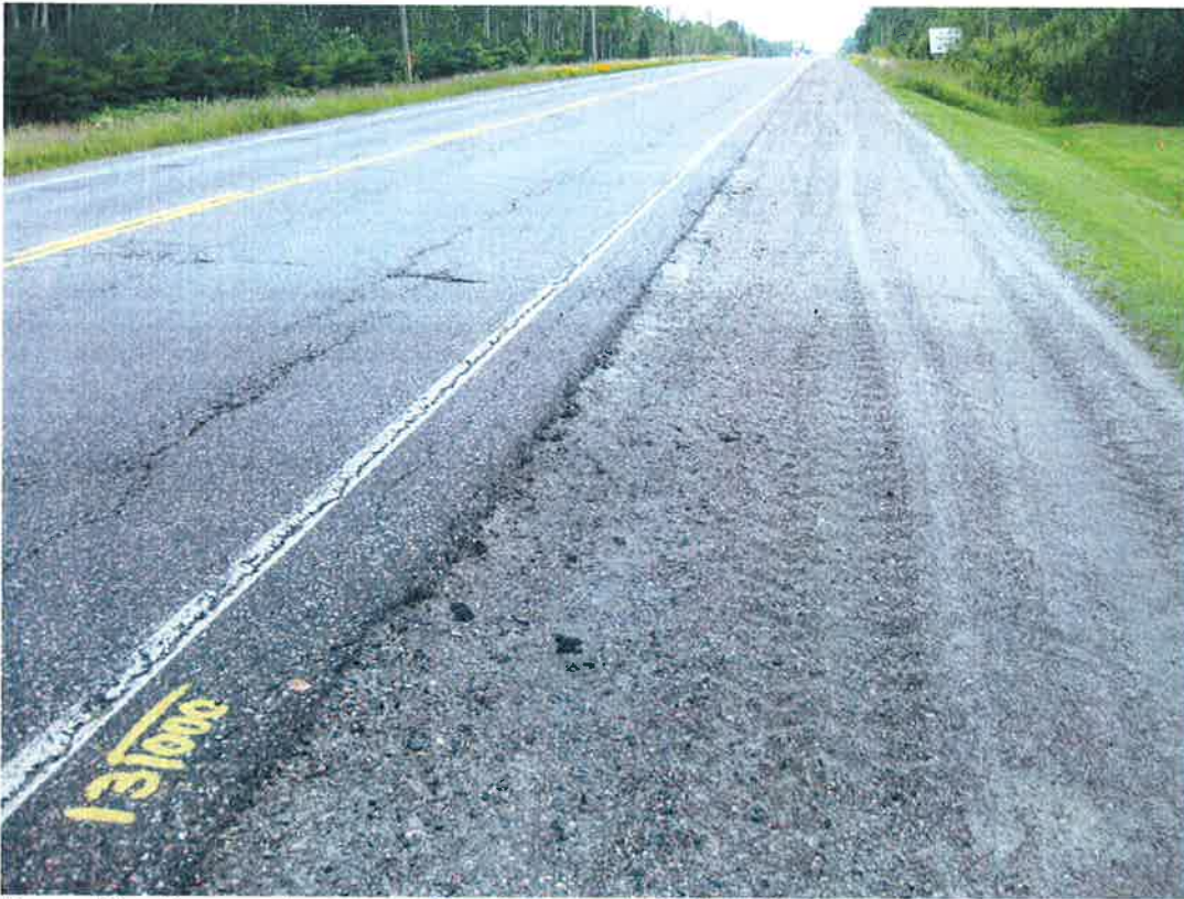
Figure D1 – Pavement cracks at Passing Lane 1, Station 13+000
