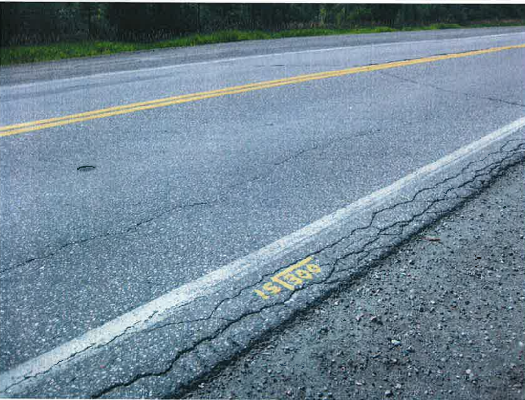
Figure D2 -Longitudinal cracks at Passing Lane 3, about Station 15+300
