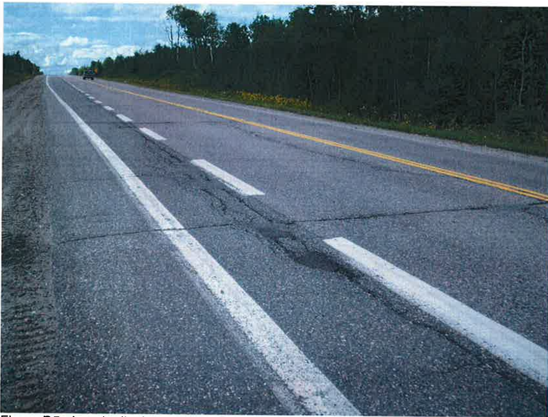
Figure D5 - Longitudinal cracking at Passing Lane 5, about Station 17+065
