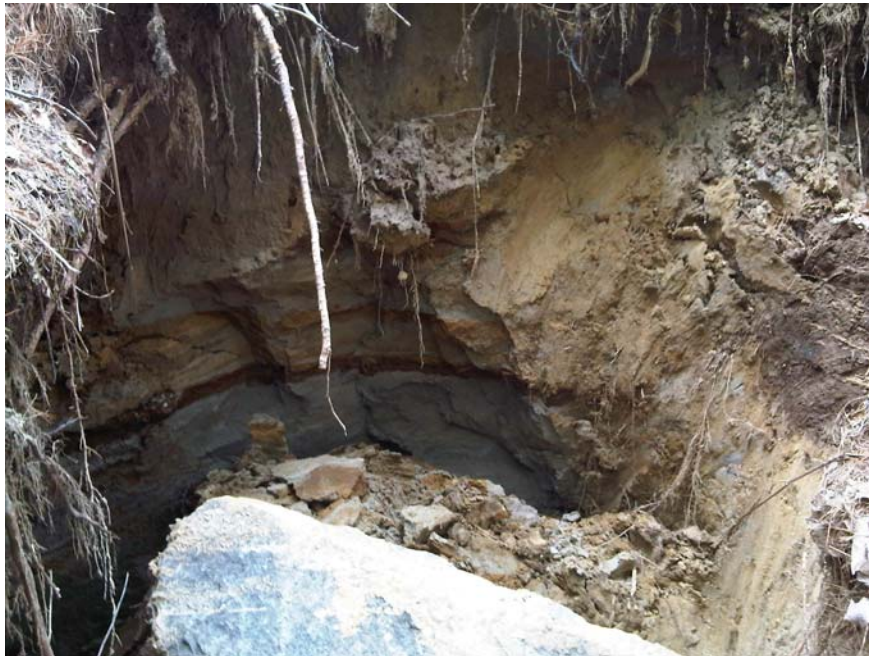
Photo 9. Sinkhole in the east embankment
