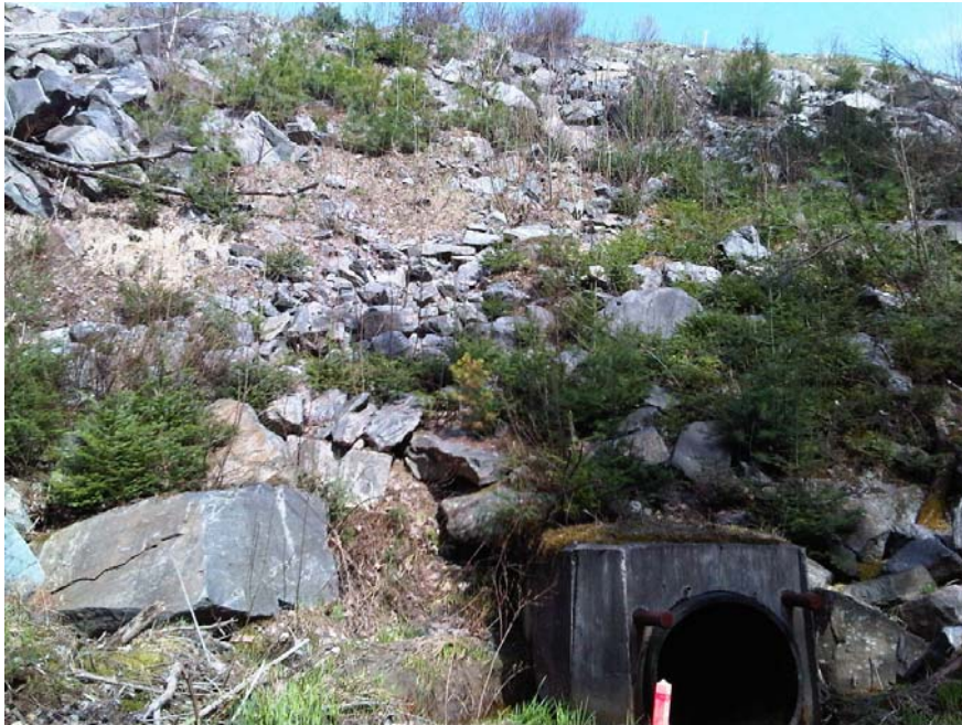
Photo 1. Inlet of the existing culvert (west side of Hwy 11)
