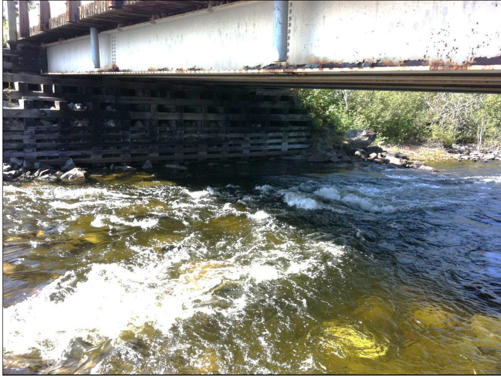
Photograph 3 – South crib abutment
