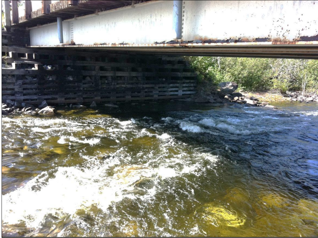
Photograph 3 – South crib abutment
