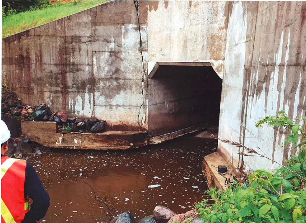
Photo 3 – Unsupported South Footing and Cracked Wingwall
