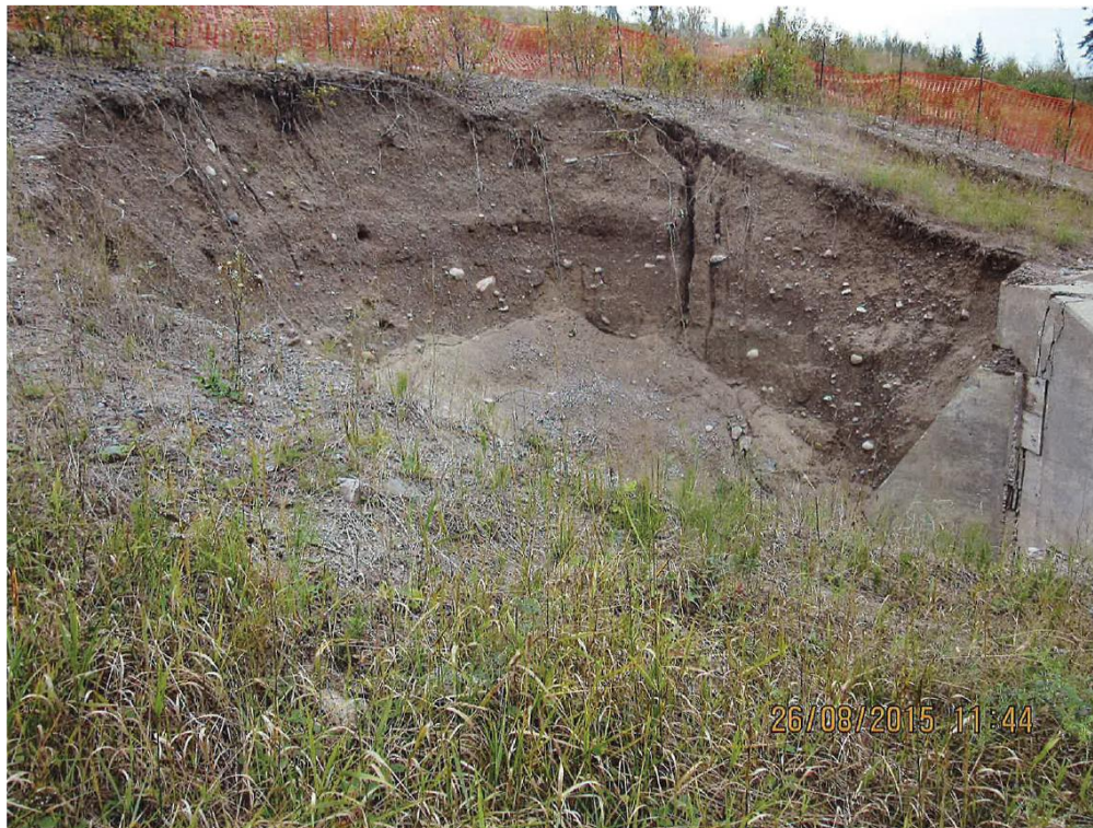
Photo 6 – Sinkhole behind Southeast Wingwall (Looking Upslope)
