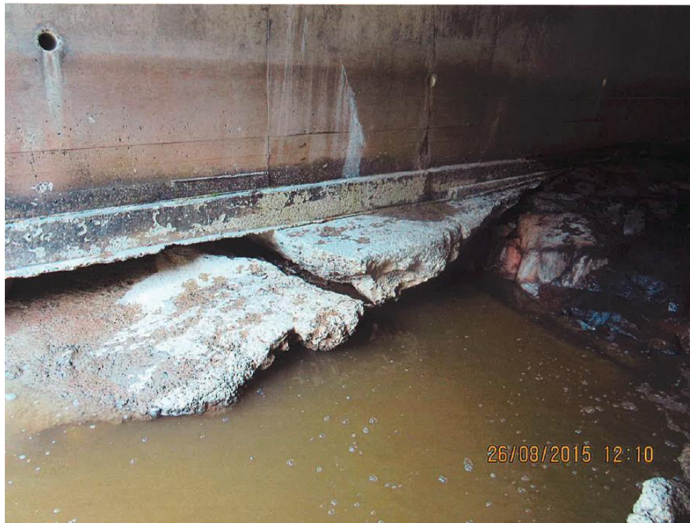
Photo 4 – Partially Supported South Footing
