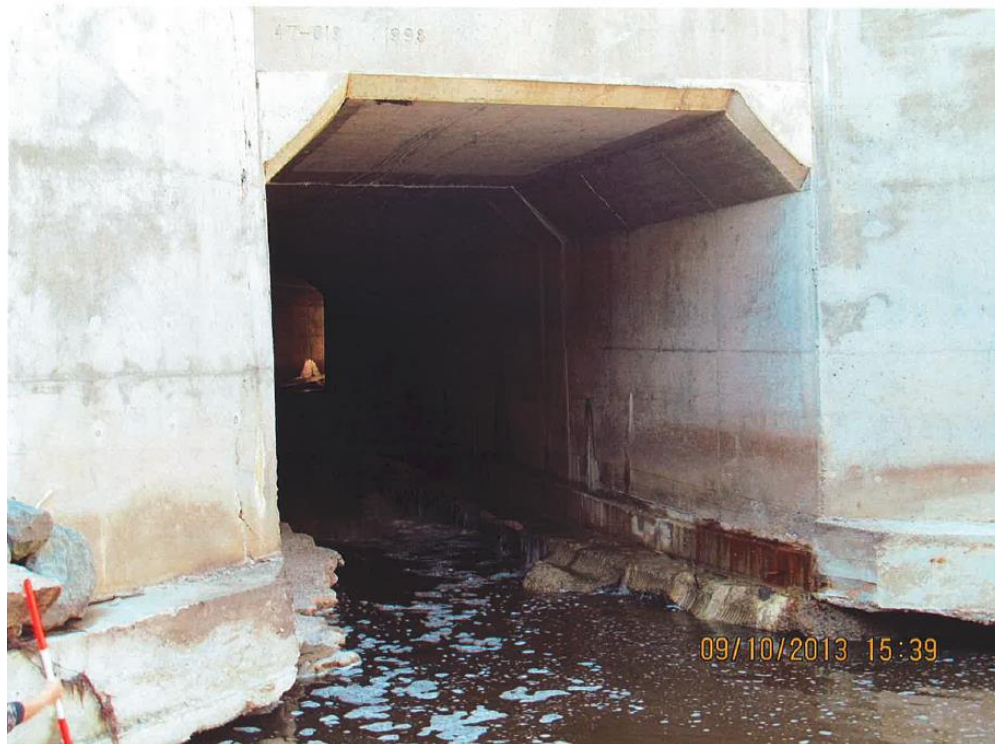
Photo 2 – Unsupported Wingwall Footings at Culvert Outlet
