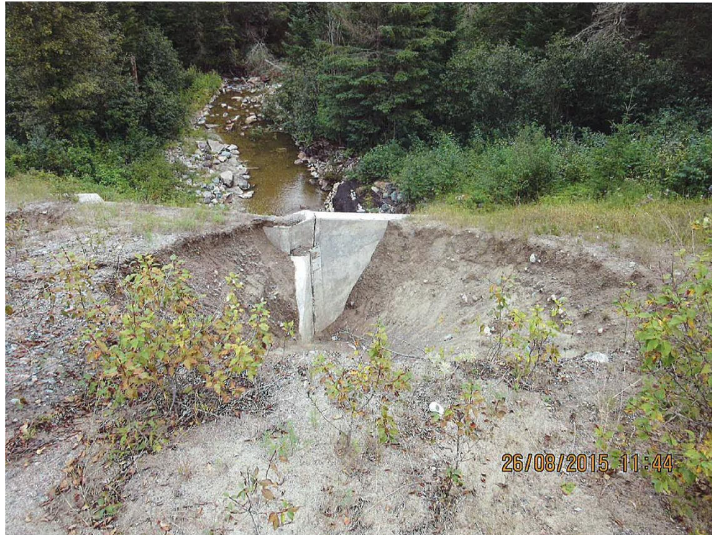
Photo 5 – Sinkhole behind Southeast Wingwall (Looking Downstream)
