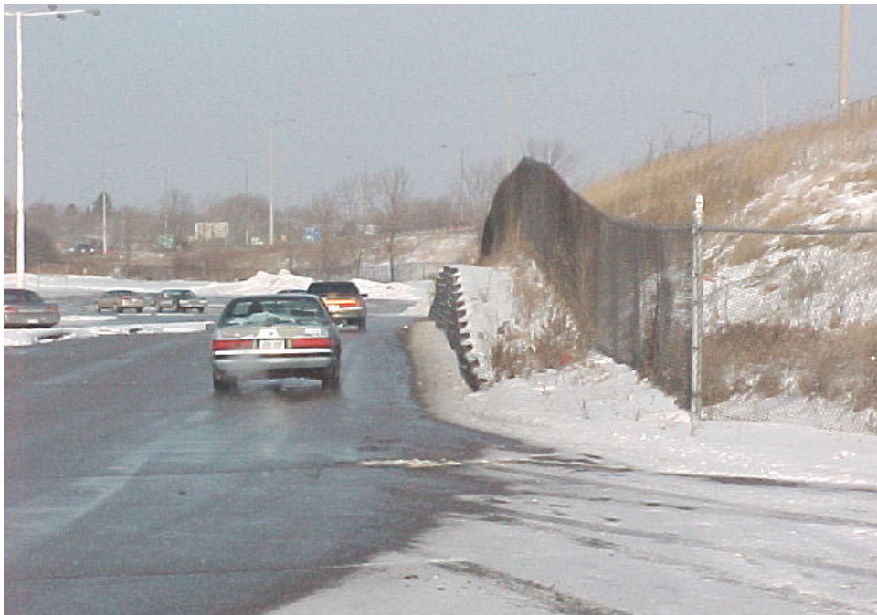
Photo 2 - Existing timber retaining wall - looking north.
