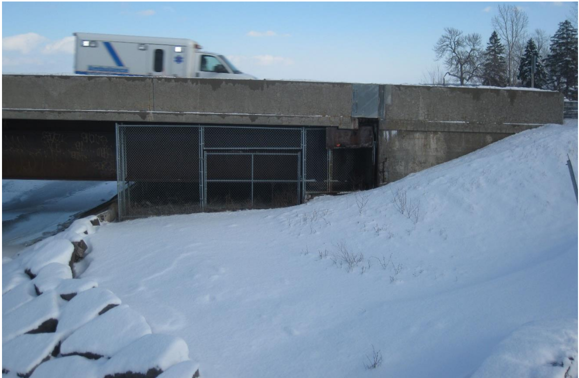
South abutment, west side, showing rock protection along shoreline
