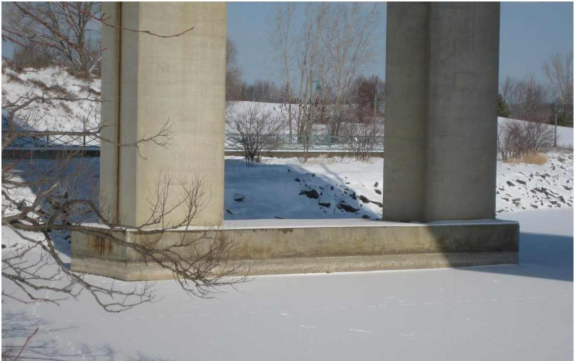
Pier adjacent to north shore, showing rock protection along shoreline
