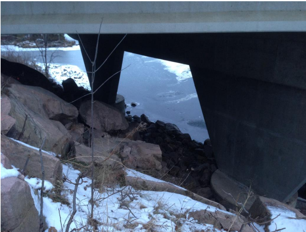
Photo 2: North Pier Showing Rip-Rap– facing east
