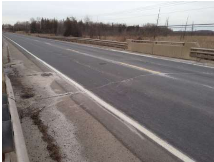
Photo 4 View Looking North Showing Pavement Distress Near Culvert
