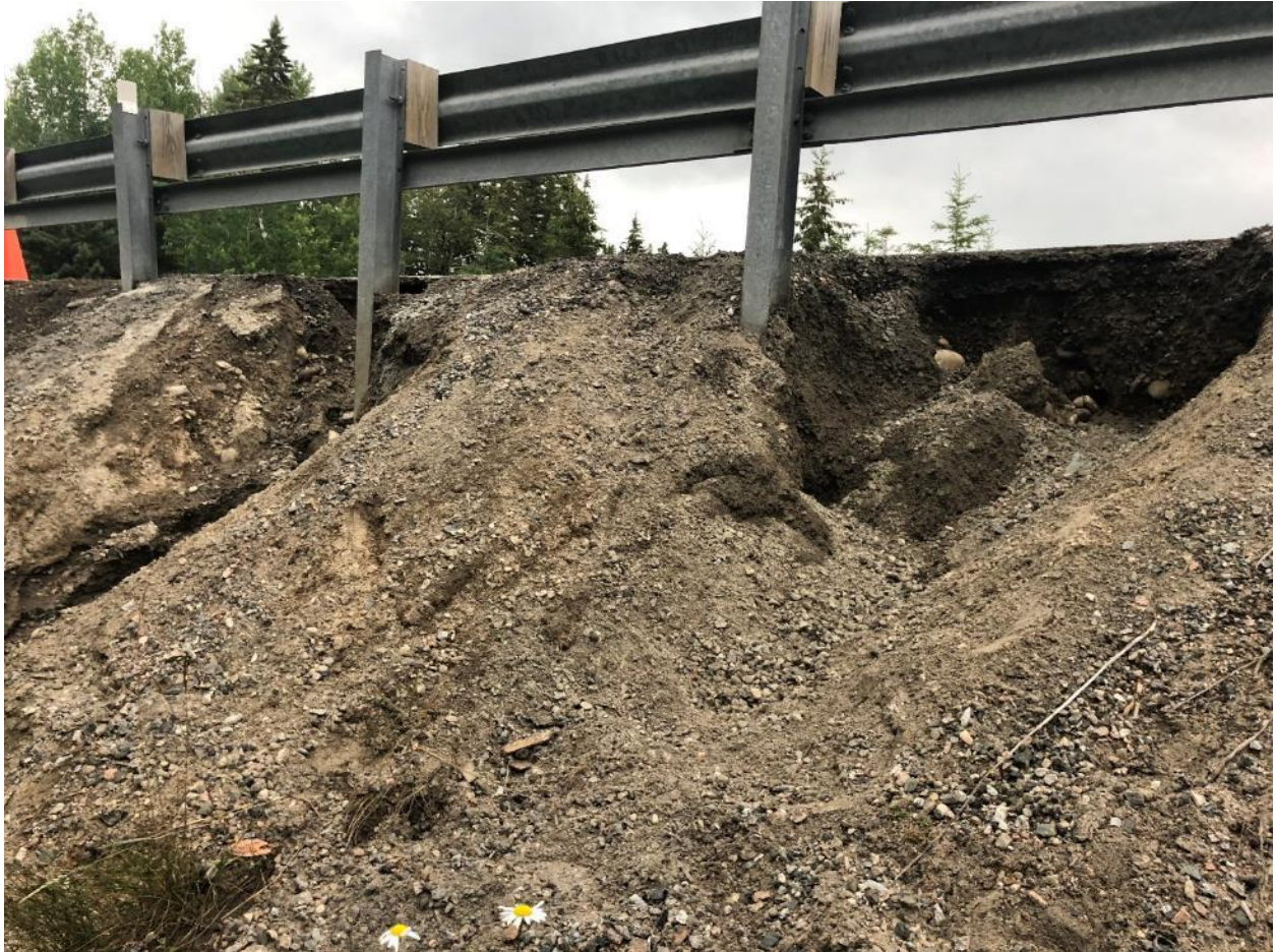
Photo C12: Close-up of erosion located northwest of culvert outlet and rockfill surface, facing north (Date taken: July 14, 2019)
