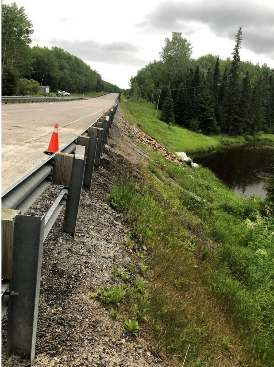
Photo C10: South side of northwest approach embankment with surficial erosion, facing southeast (Date taken: July 14, 2019)
