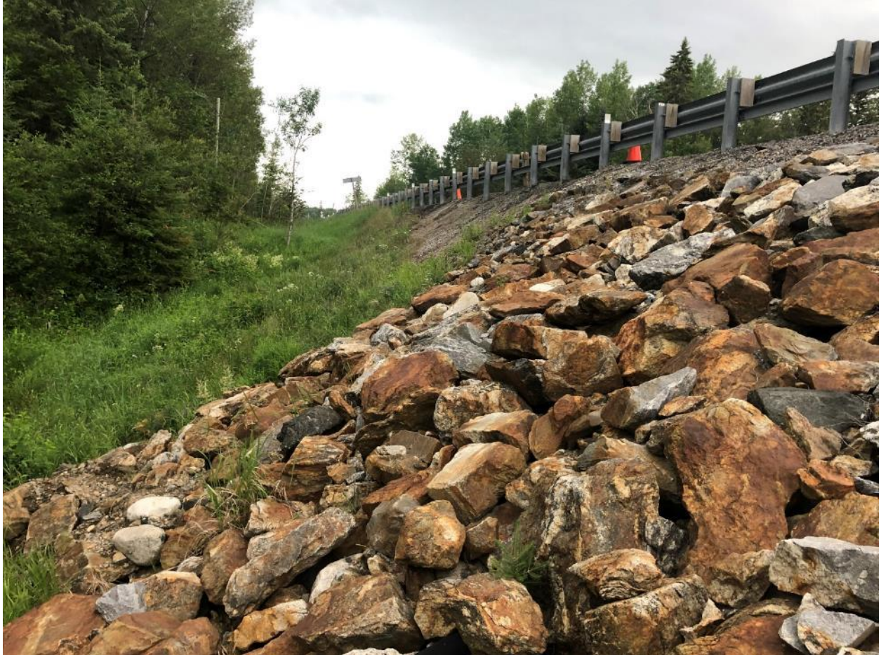
Photo C8: South side of northwest approach embankment with rockfill surface, facing northwest
