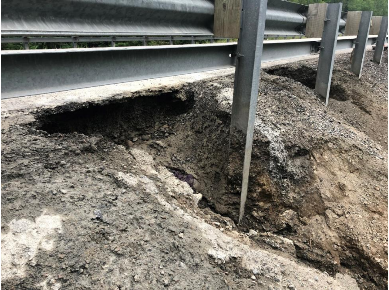
Photo C13: Close-up of erosion located northwest of culvert outlet and rockfill surface, facing east (Date taken: July 14, 2019)
