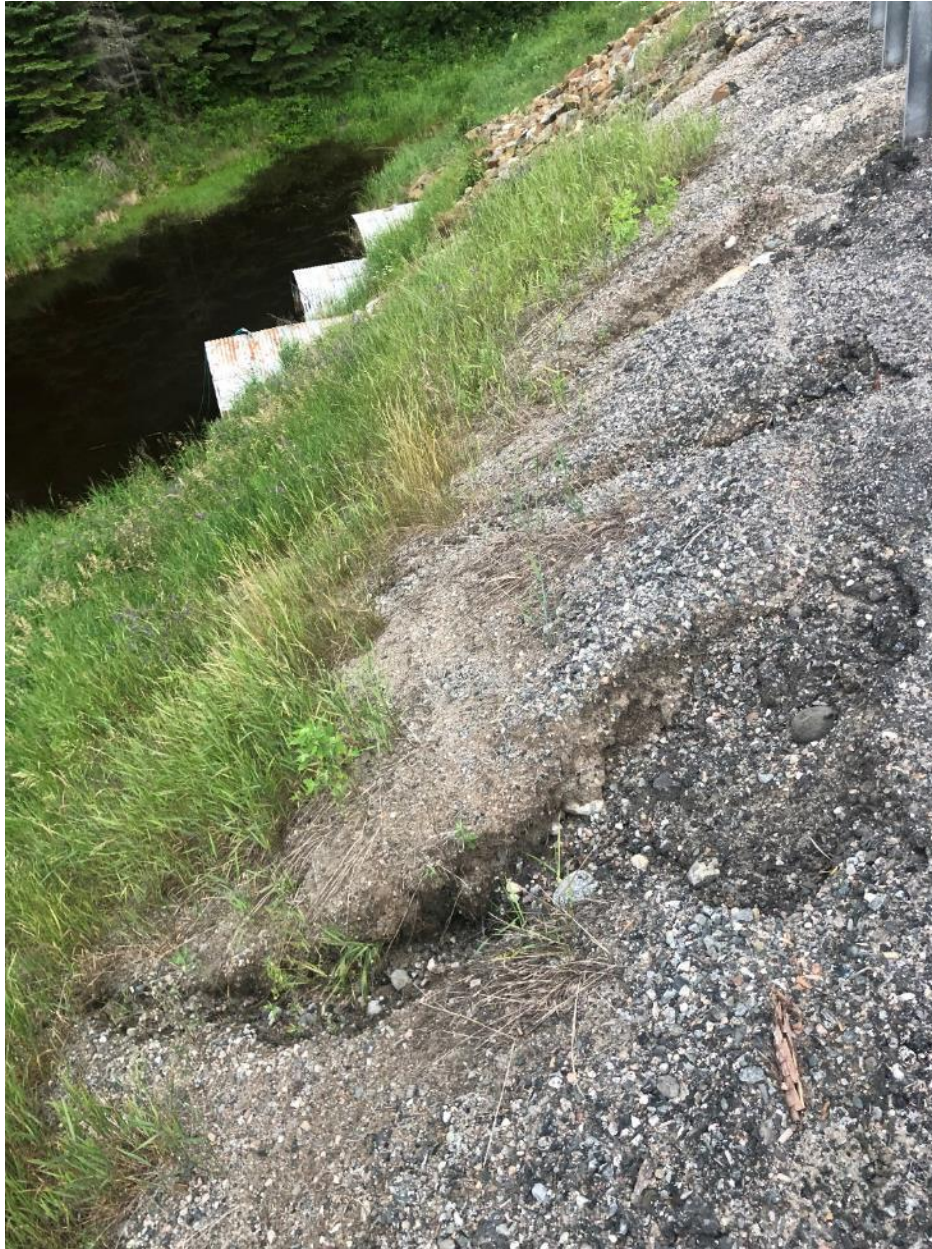
Photo C14: Surficial erosion of granular shoulder on south side of embankment, southeast of culvert outlet, facing northwest (Date taken: July 14, 2019)
