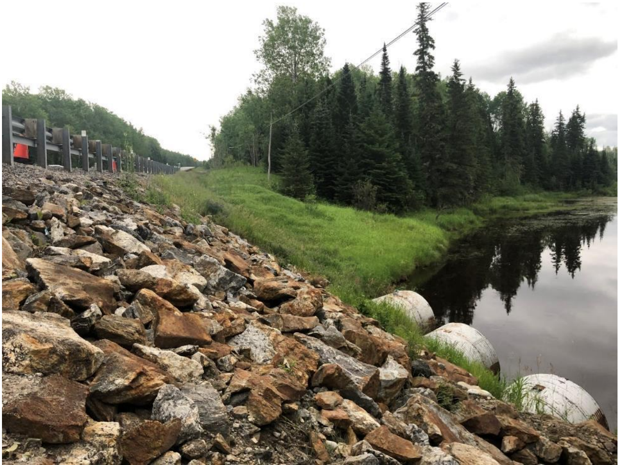
Photo C6: Culvert outlet and rockfill surface on south side of embankment, facing southeast approach (Date taken: July 14, 2019)
