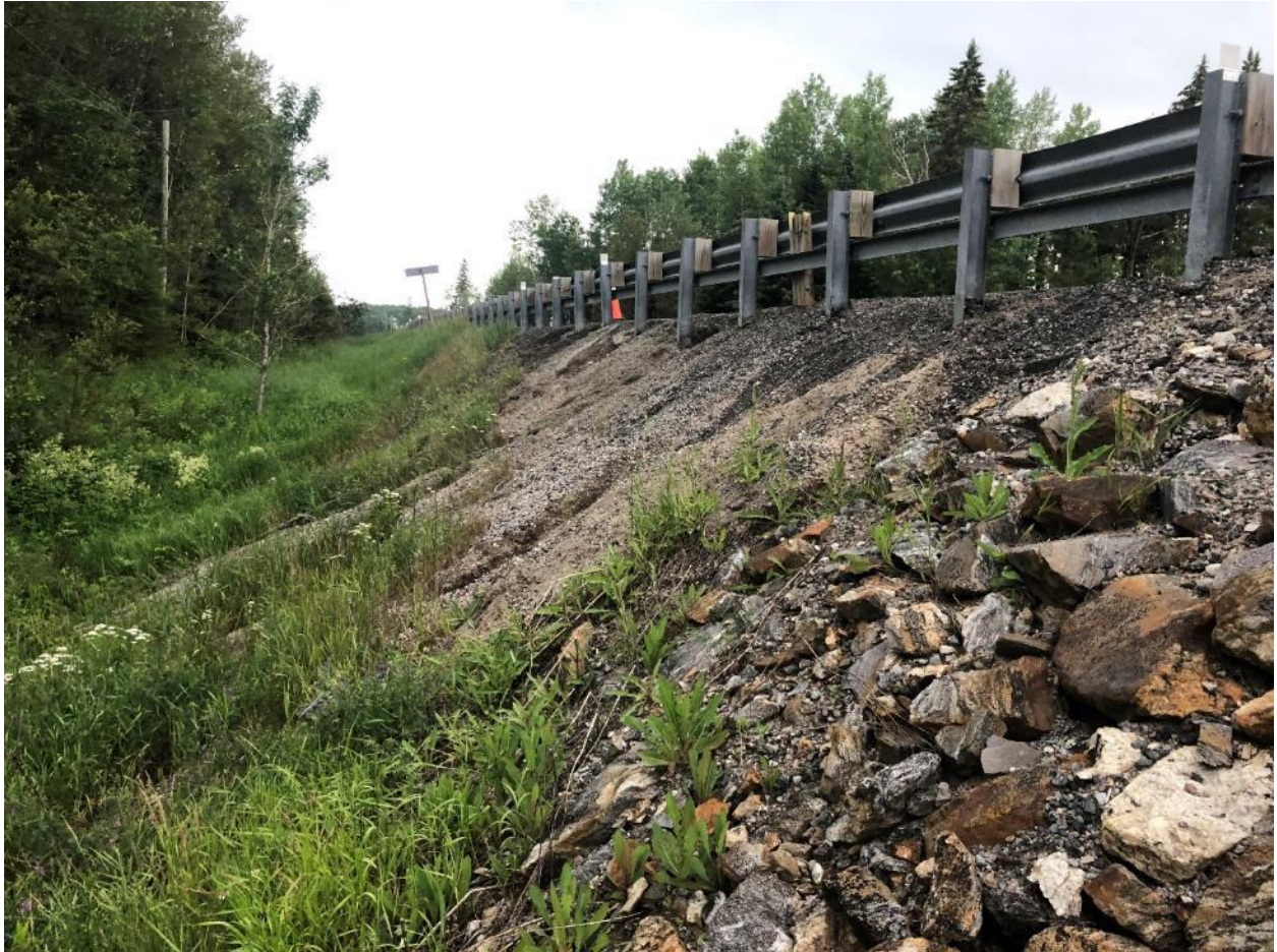
Photo C9: South side of northwest approach embankment with surficial erosion, facing northwest
