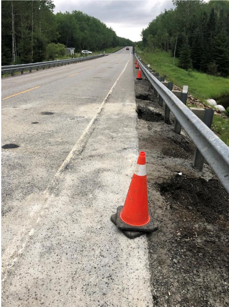
Photo C11: Surficial erosion of granular shoulder on south side of embankment, facing southeast (Date taken: July 14, 2019)
