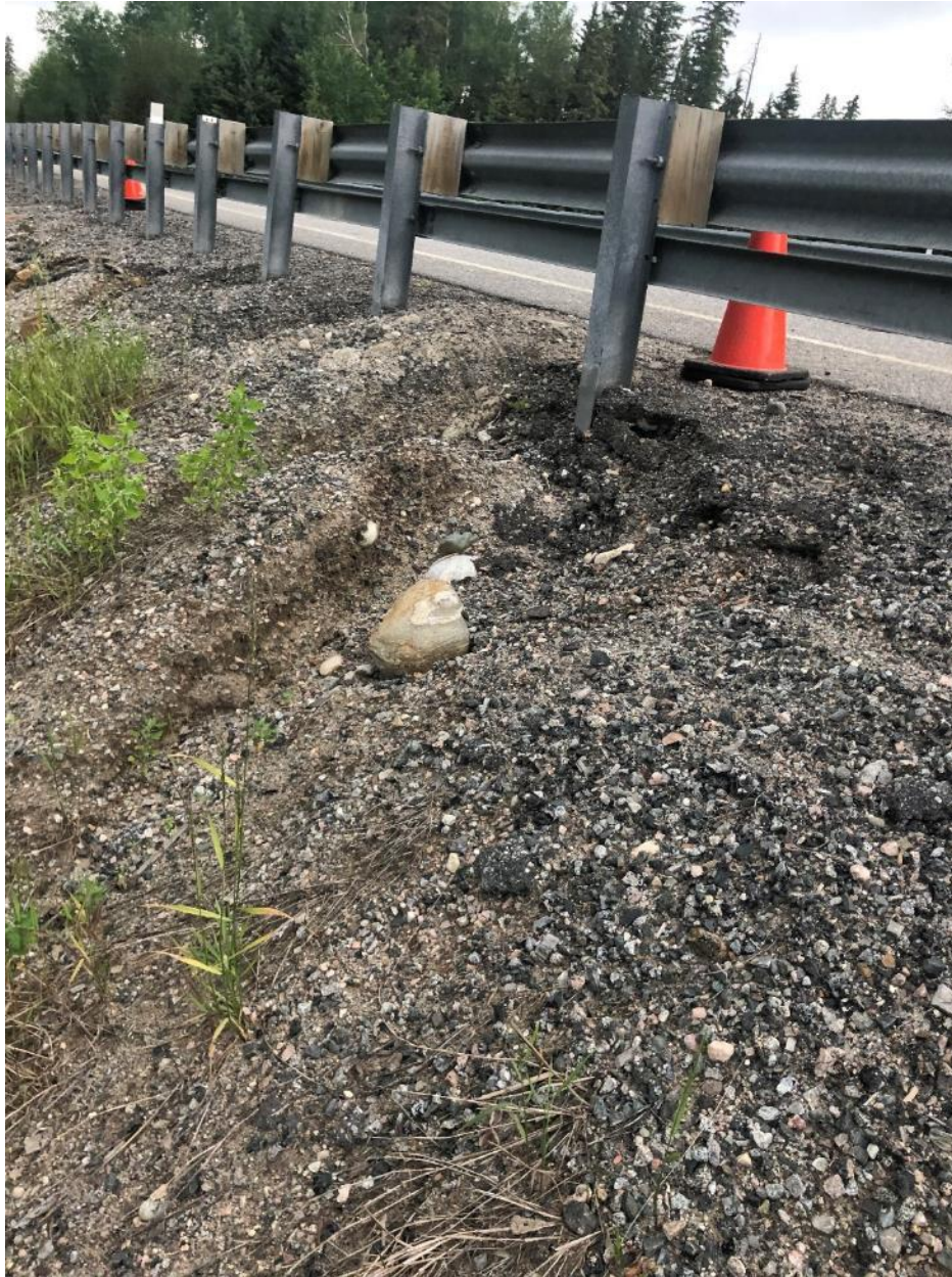
Photo C15: Close-up of erosion located southeast of culvert outlet and rockfill surface, facing north (Date taken: July 14, 2019)
