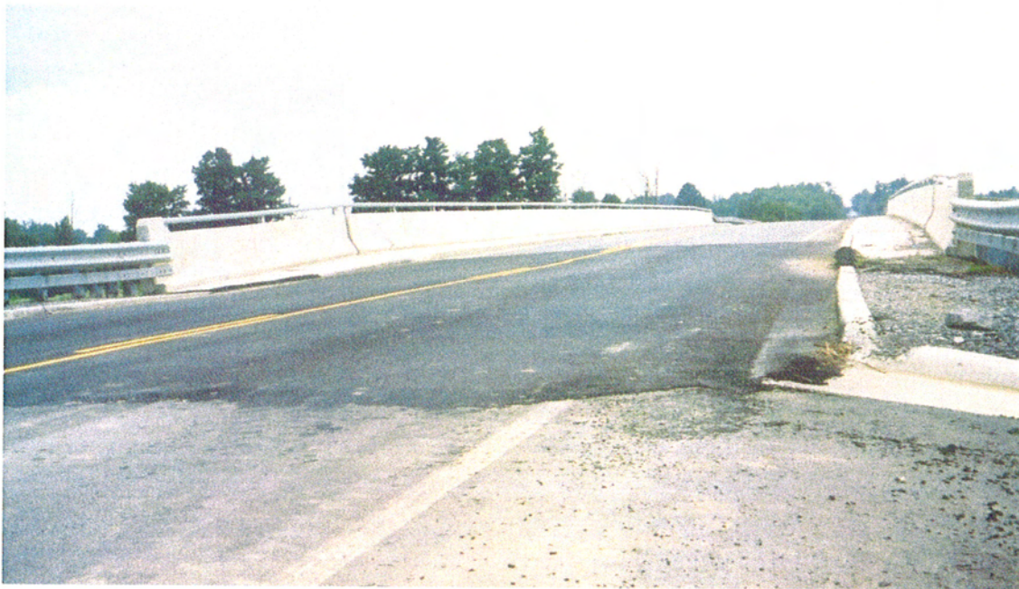
Figure J-3 Asphalt Patching Adjacent to North Abutment (Photograph Date : August 01, 2003)
