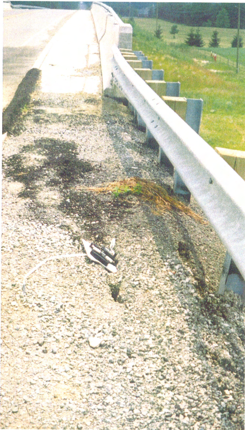
Figure J-5 Crack Along North-West Shoulder (Photograph Date : August 01, 2003)
