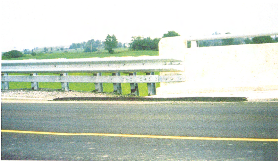
Figure J-4 Sealing of Cracks Adjacent to Asphalt Patching Near North Abutment (Photograph Date : August 01, 2003)
