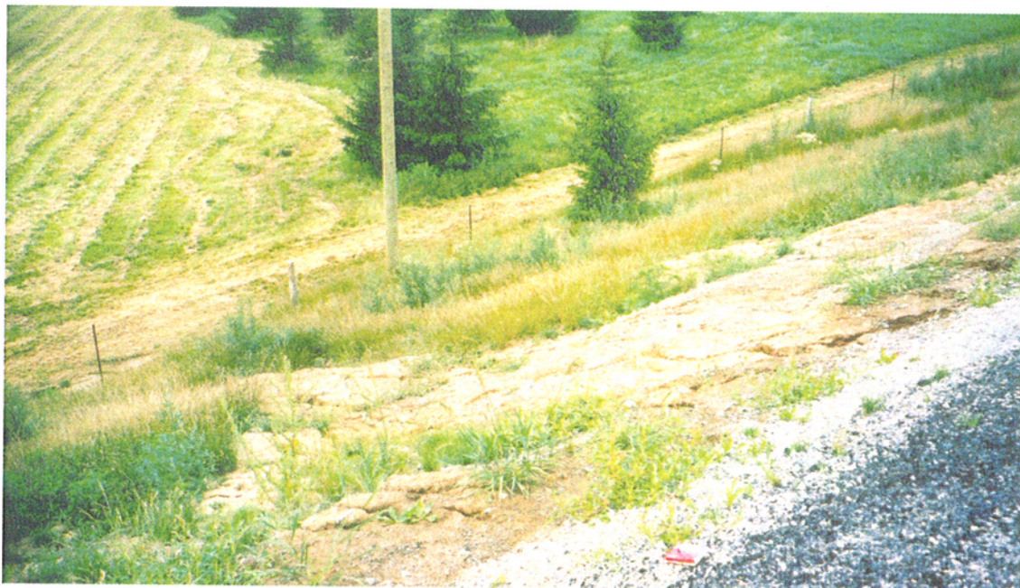
Figure J-7 Slumping and Erosion Along West Embankment Slope, South of South Abutment (Photograph Date : August 01, 2003)
