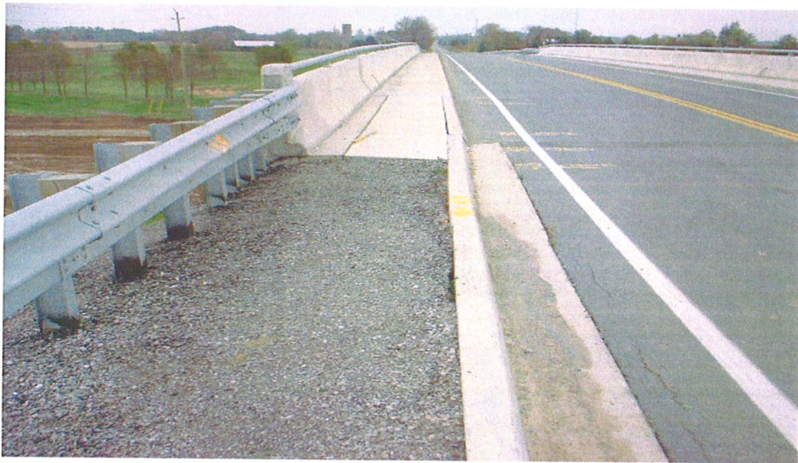
Figure J-6 South of South Abutment, West Shoulder Area, Various Cracks (Photograph Date : October 18, 2003)
