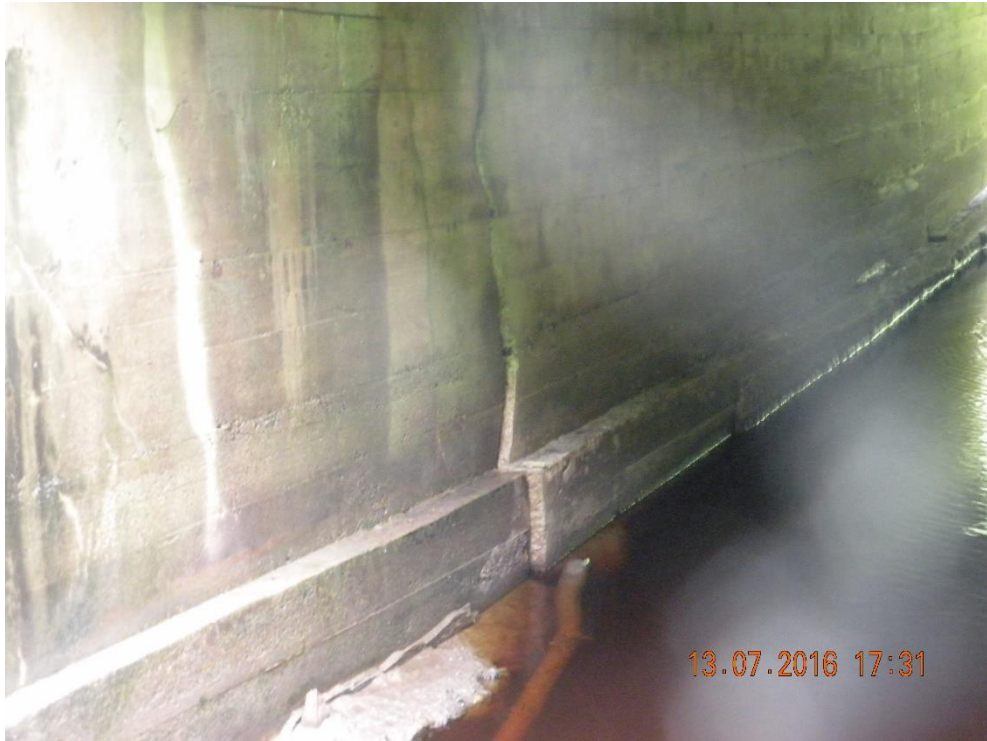
Photo 5: Cracking and push-out of culvert wall
