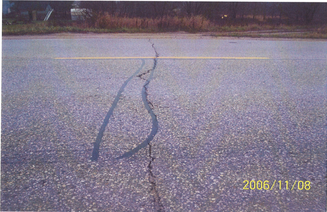
Typical Transverse Crack in Varney Section
