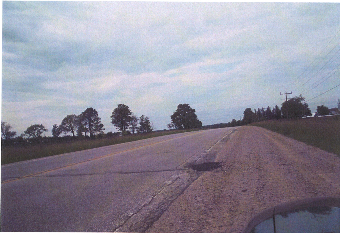
Severe Transverse Crack, Highway 6
