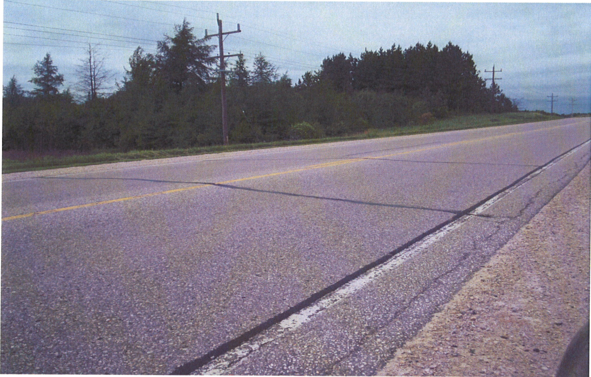
Slight, Throughout Coarse Aggregate Loss
