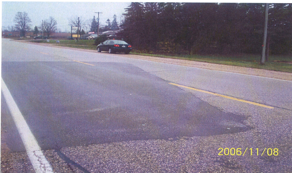
New Patch at Sta. 28+100, Varney Section
