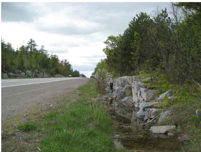
← Photo 3 Bedrock cut on north side of Highway 17 noting pool of water generated from groundwater seep (Seep 1). Photo taken facing west.
