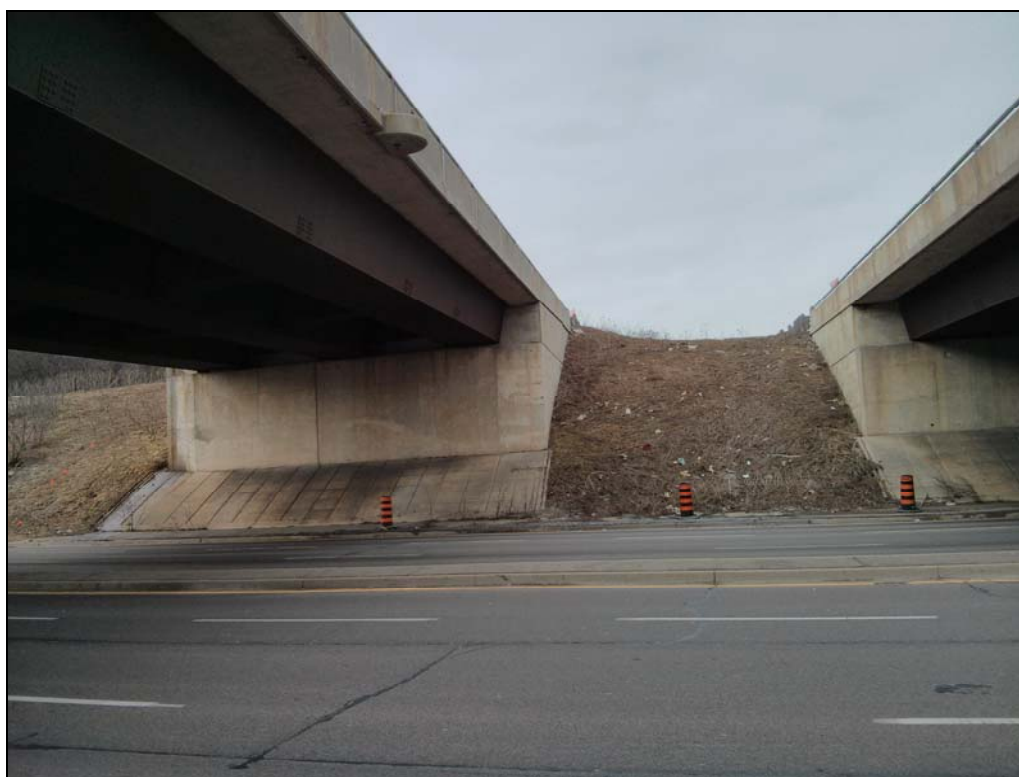
Photograph 2: On the right - west abutment of the structure carrying the EB QEW at Ford Drive.
