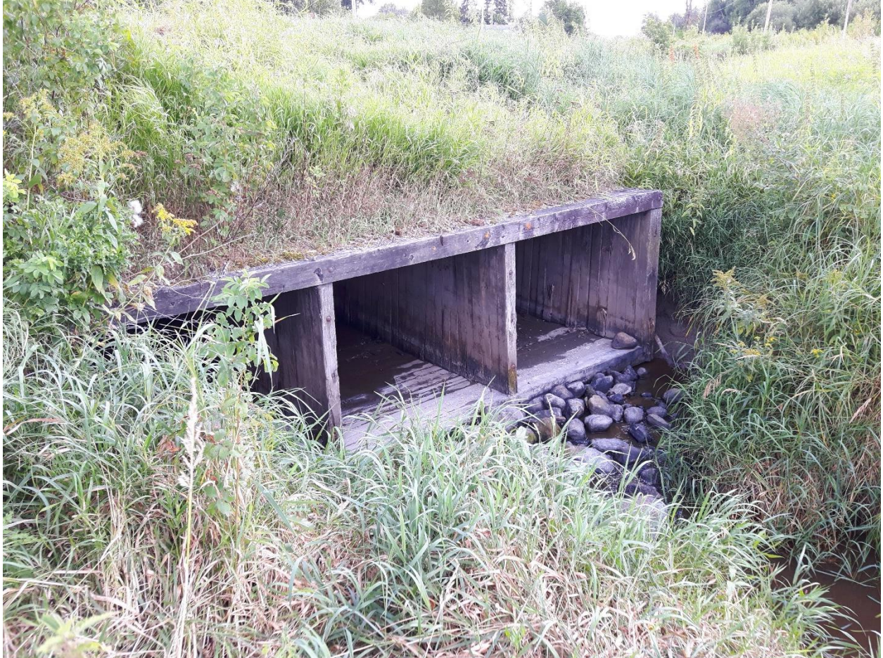
Photo 1: Looking south at north end of existing culvert.
