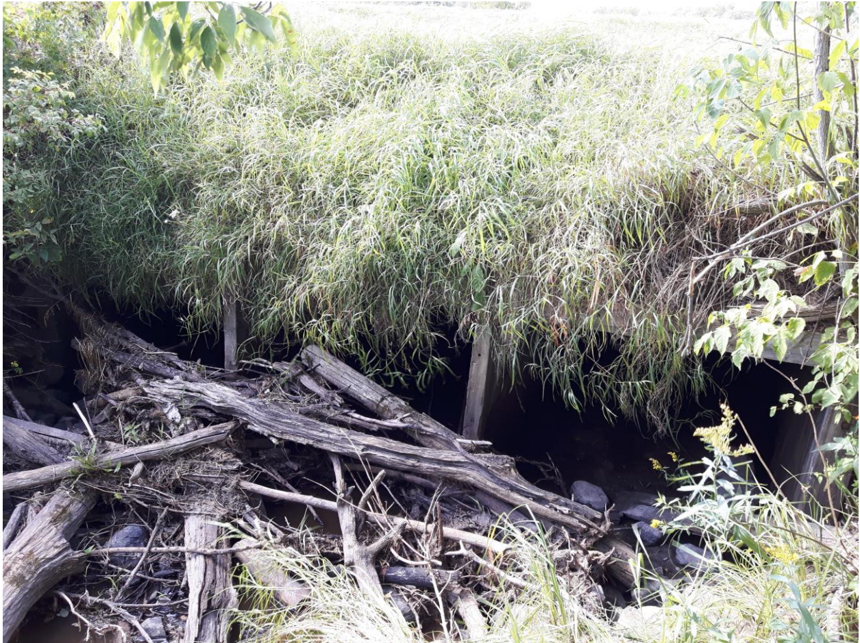
Photo 2: Wood debris accumulation at south end of existing culvert.
