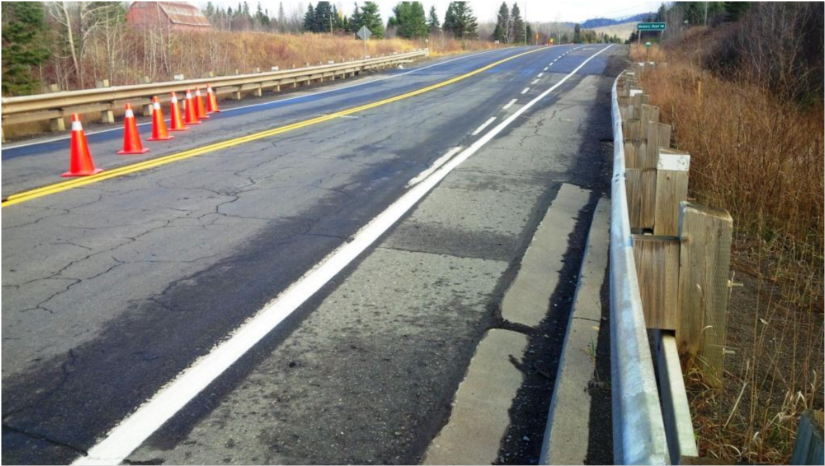
Photograph 9 – Settlements at North Approach – Leaning Guide Rail
