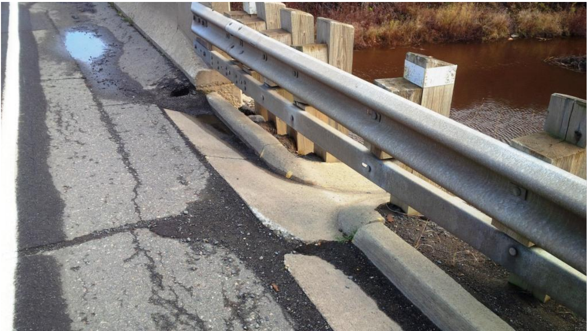
Photograph 8 – Settlements at Southeast Wingwall
