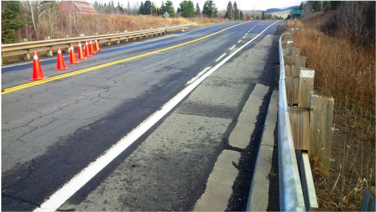
Photograph 9 – Settlements at North Approach – Leaning Guide Rail
